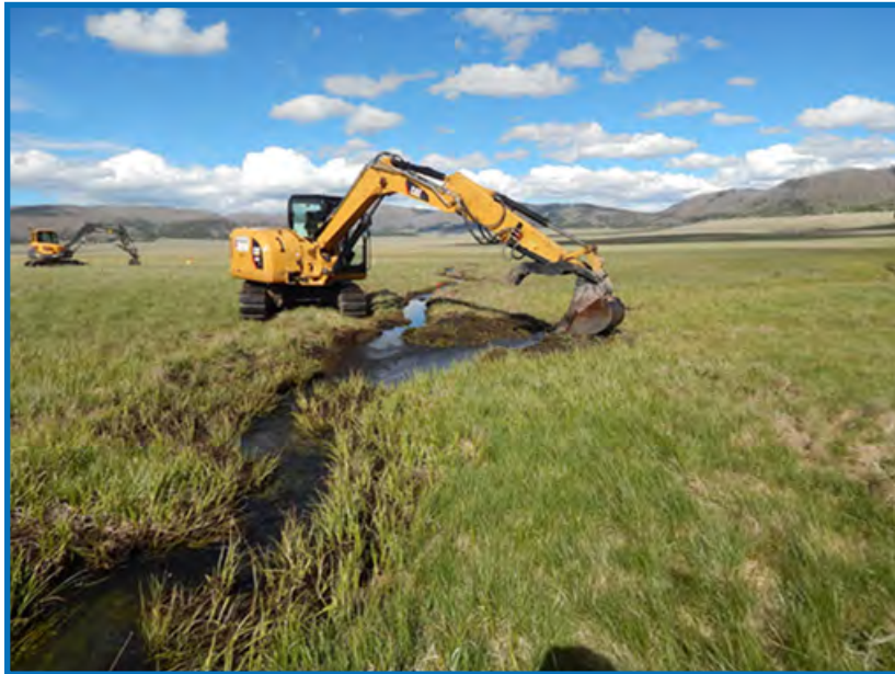
Subcontractor Keystone Restoration Ecology creating an excavator plug that will re-direct and spread water from the channel into historic wetlands.
