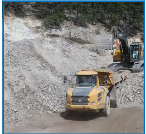
2019 - Loading waste rock containing elevated levels of lead at West Cut.
