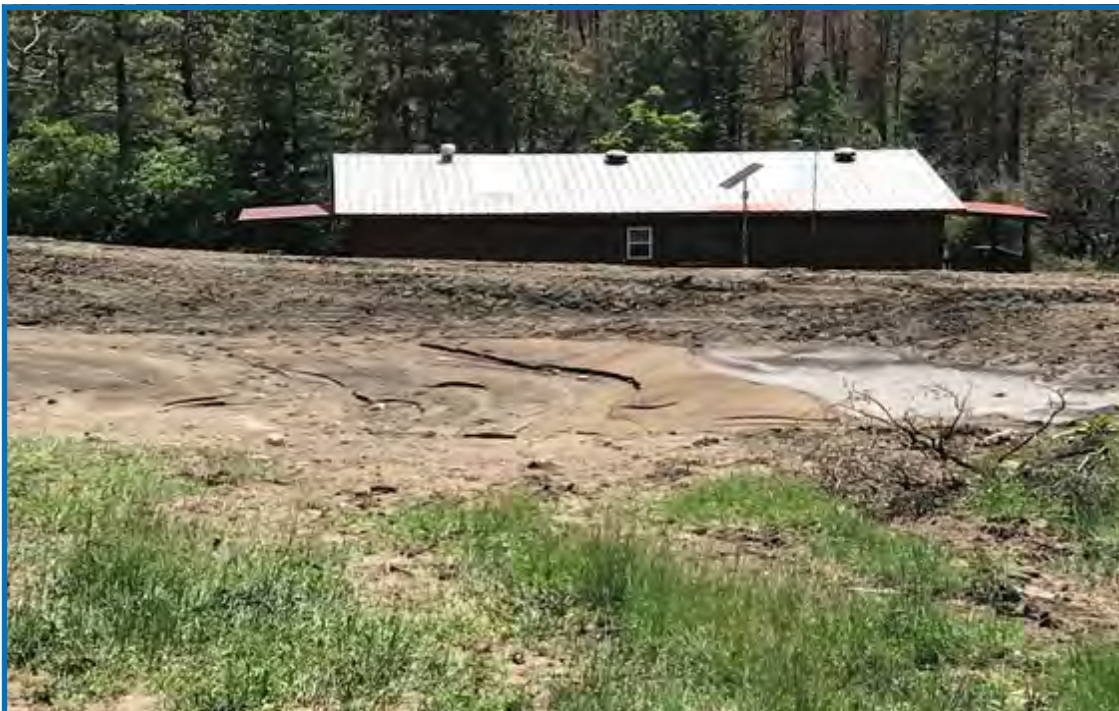
Photo above shows a structure in danger of being overcome with debris and sediment. Photo below shows diversion constructed to protect the structure from debris and sediment. The debris upstream was removed offsite and the diversion was reseeded. Picture shows the amount of sediment that has been diverted from the structure.
