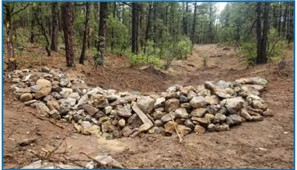
Rock and brush dam built in previous year.
