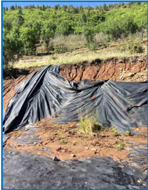
Large amounts of erosion control fabric in Curtis Canyon was removed .
