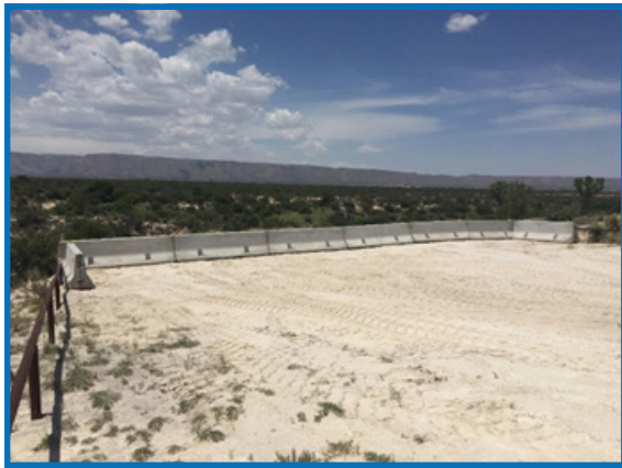
2019 - Ladder Hole recreational parking area – Black River, New Mexico.
