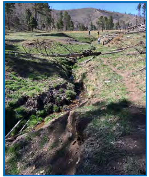
Anan Creek restoration to begin in fiscal year 2020; headcut repair and other grade control treatments to arrest further channelization will be implemented in these areas.
