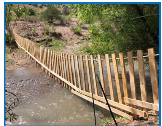
Bottom photo: Side view of recently completed Gila River water gap.
