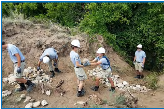
Installing check dams on upland drainages, headcuts, and gullies near the Rio Bonito.
