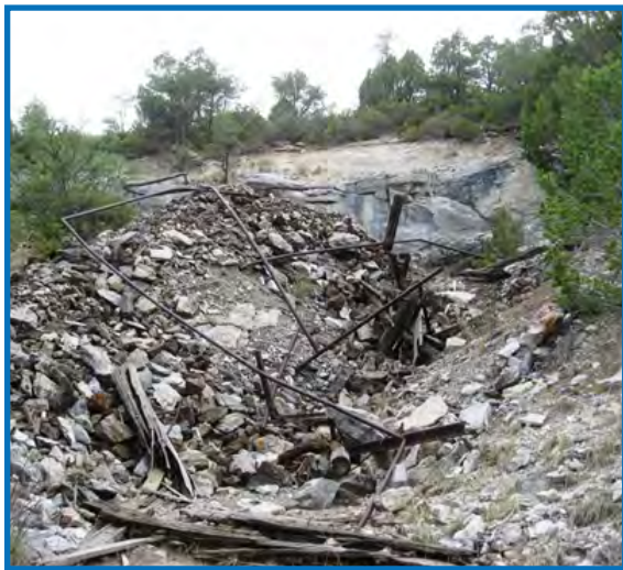
2018 - Waste piles at the West Cut of Royal John Mine before cleanup.
