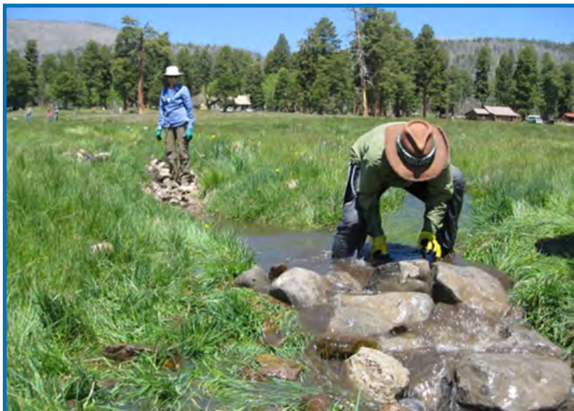
Subcontractor Keystone Restoration Ecology creating an excavator plug that will re-direct and spread water from the channel into historic wetlands.
