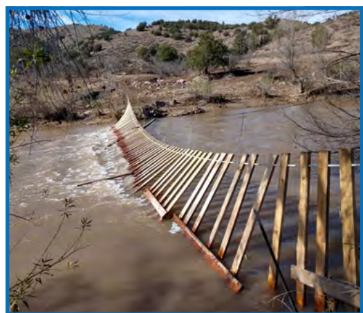
Side view of Gila River water gap functioning following November storm.
