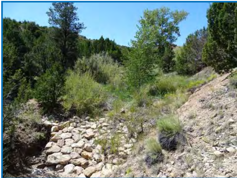
Figure 5.3 from Rio Embudo WBP, an example of a "perched wetland" with potential for retaining sediment. This example on BLM land was stabilized in 2013. The WBP identifies several locations where similar work would have the double benefit of enhancing small wetlands and preventing sediment loading to the Rio Embudo.
