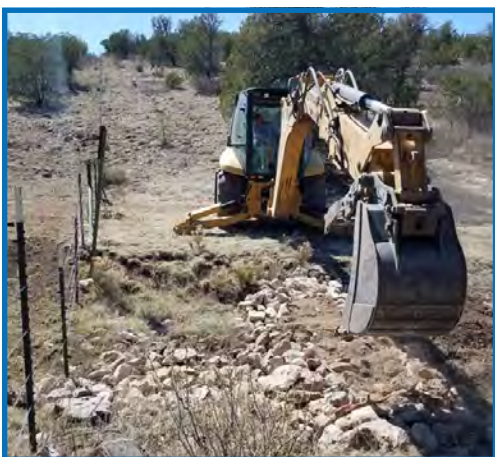
Installing Check Dams on upland Drainages, Headcuts, and Gullies on Fort Stanton Snowy River Cave National Conservation Area.
