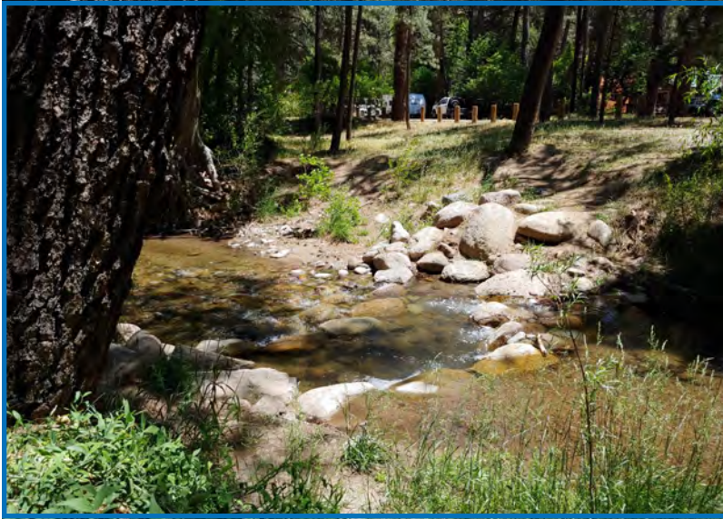
Cross-vane structure with newly formed scour pool and willow pole plantings at Two Rivers Park, June 2019.
