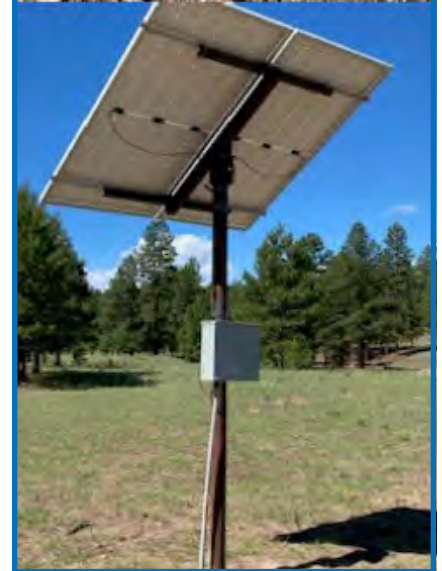
New solar well (Adair Well) to provide alternate water source to Adair Spring.
