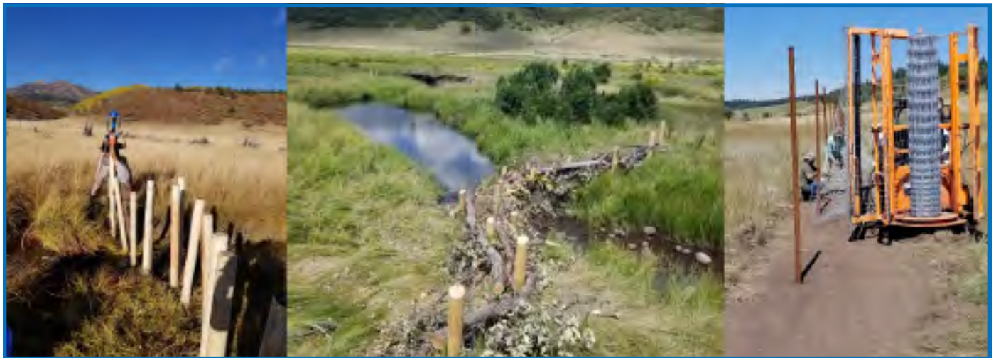
Photo montage; Sargent Wildlife Management Area with post assisted log structures, beaver dam analog, and enclosure fencing.
