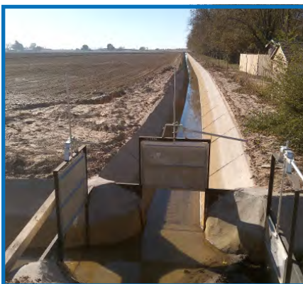
Photo left; Lined Ditches and Structures for Water Control installed through the NWQI.
