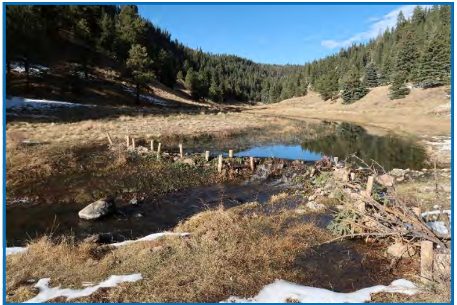
San Antonio Creek Restoration project - 12 additional beaver dam analogues and 15 log baffles were installed.
