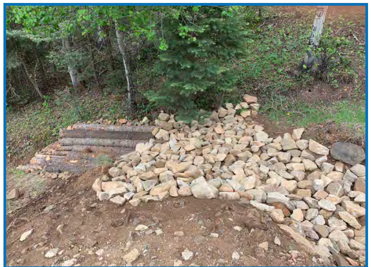
An example erosion prevention treatment of the small ephemeral channel adjacent to the road.
