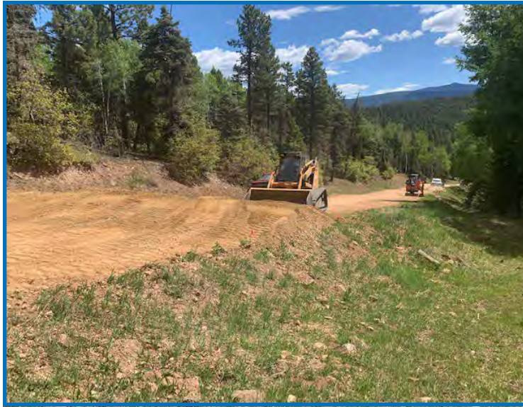
An example erosion prevention treatment of the small ephemeral channel adjacent to the road.
