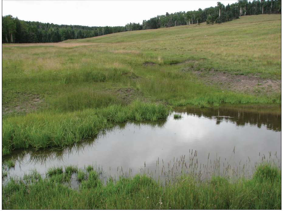
Figure 51. Placement of this small stock tank shows drying of wetland vegetation above and below the tank, an incised channel below the tank spill way, and a headcut that is migrating upstream.
