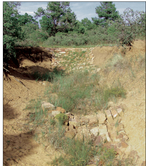
Figure 76. This rock rundown was constructed in an arid environment; however, the same design and construction principles would apply for a slope wetland stabilization treatment.
