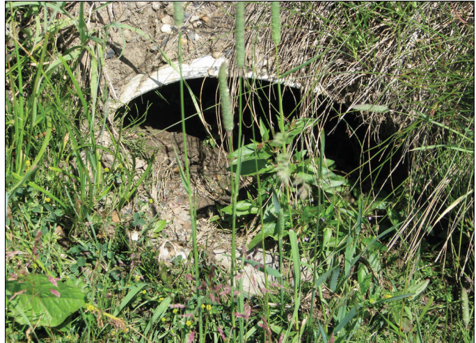
Figure 42. A blocked culvert will deprive downslope wetlands of water by diverting flow to another location.
