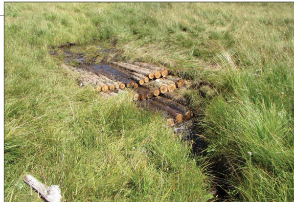
Figure 74. The log and fabric step falls schematic shows the detail of material placement (Zeedyk and Clothier, 2009). The log step fall in this photograph was built by volunteers in the Grassy Creek slope wetlands.
