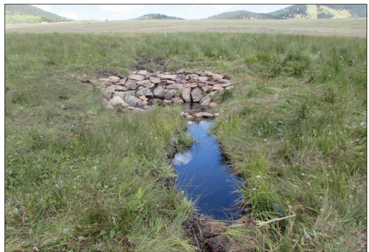
Figure 73 is a Zuni bowl constructed by volunteers in the Grassy Creek slope wetlands in the Comanche Creek Watershed. The one rock dam can be seen in the photograph. Below the pool is a sod plug which is helping to slow water flow through the incised channel below the headcut and rewet the slope wetland surface.
