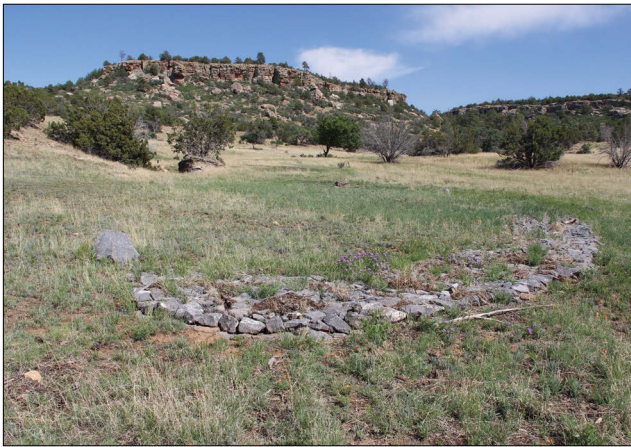
Figure 57. The schematic shows proper placement of the media luna structure and the subsequent photographs show a newly constructed media luna and the same media luna as recovery progressed at a restoration site near Wagon Mound, New Mexico.
