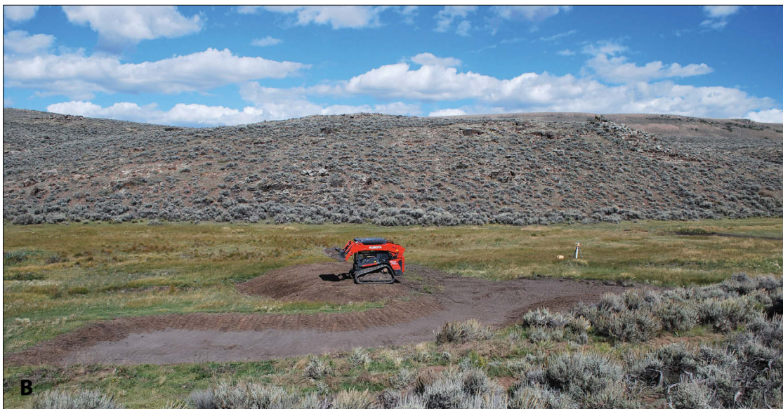
Figure 55 A. The schematic shows a plug and pond design with one bay flooded. Figure 55 B shows the implementation of the plug and pond treatment in a slope wetland complex near Gunnison, Colorado
