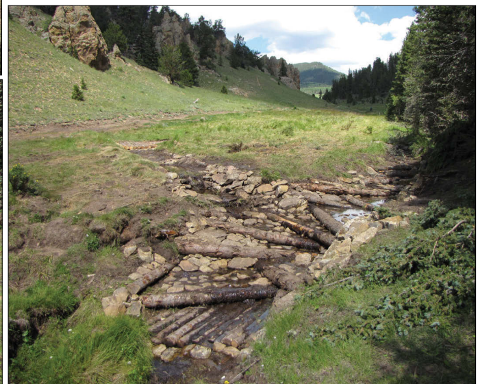
Figure 53. A large headcut is draining this slope wetland. Left alone, this headcut will continue to erode away at the wetland as the headcut moves upslope. In this situation, stabilization is necessary before any other restoration work could be effective. Construction of the log and rock step falls stabilizes the wetland complex and has positive effects in increasing slope wetland function both upslope and downslope of the stabilization site.
