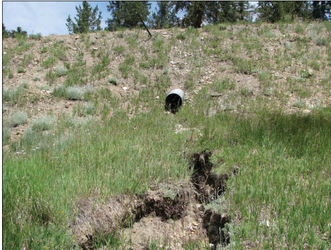
Figure 41. The outflow of this culvert is causing erosion at the top of a slope wetland. Armoring the drain would help mitigate this condition. Culverts installed too deeply initiate headcutting on the upstream side of the road as well.
