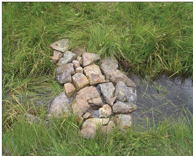
Figure 63. A one rock dam has been used in an incised channel to slow and raise the water level upvalley in order to reconnect the water with the wetland surface.
