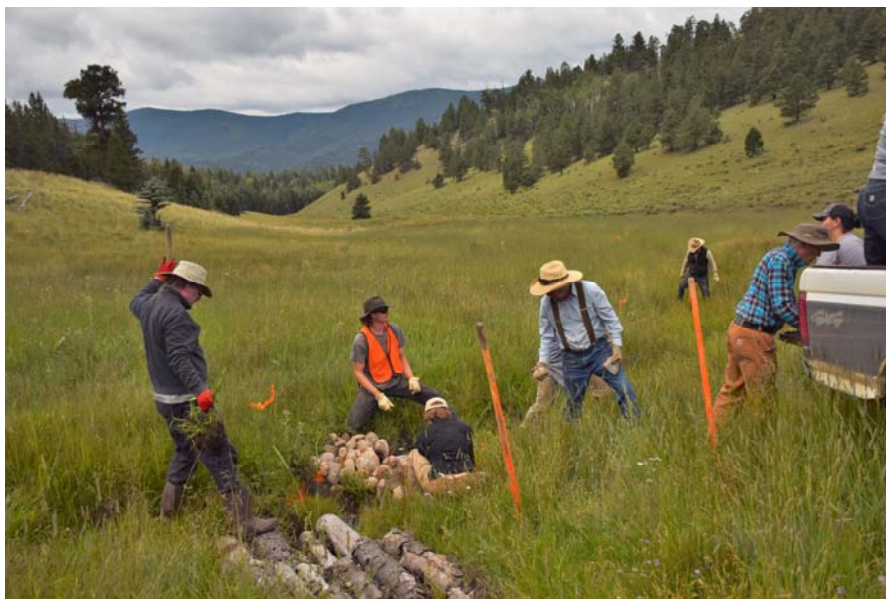
Quivira Coalition building one-rock dams to capture sediment and raise water table in slope wetlands in the Comanche Creek Watershed
