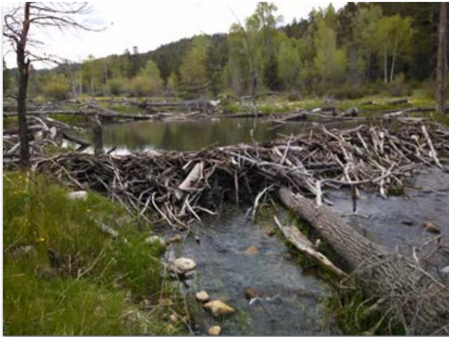
Beaver dam on El Rito Creek in the Carson National Forest, Northern NM
