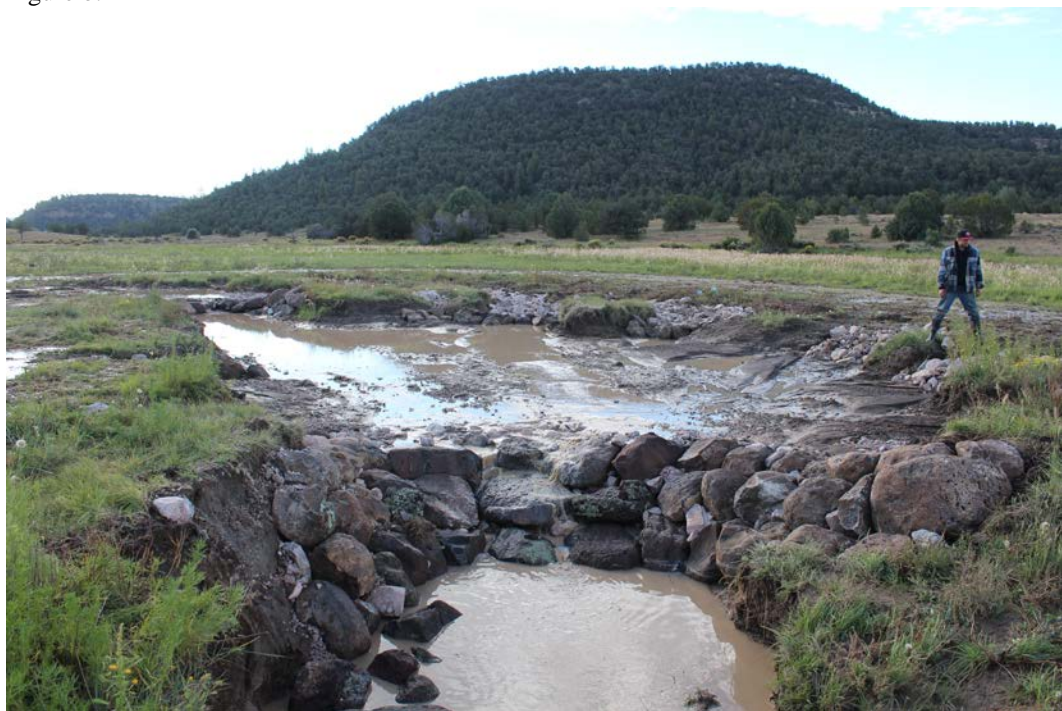
Figure c. This photo shows the use of a combination of innovative structures to arrest a large headcut and slow and distribute flow across the floodplain. In the background, a Media Luna structure spreads the flow and reduces flow velocities above the headcut. A number of Rock Rundowns armor small cuts around the main incised channel. A Zuni Bowl structure is used to heal low headcuts up to two feet high. Zuni Bowls harden the base of the cut to stop scour and undercutting; protect the face of the headcut from drying, sloughing and frost heave; and conserve moisture for enhanced plant growth. The rocks capture sediments, debris, seeds, and plant propagules, and act as rock mulch that protects young plants. They are frequently used in conjunction with one-rock dams.
