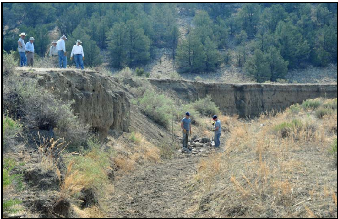
Figure 25. National Wild Turkey Federation volunteers building structures to induce meandering in Reach 7 (the critically incised portion of Cebolla Canyon downstream of the Cebolla Springs wetland) - Summer 2013.
