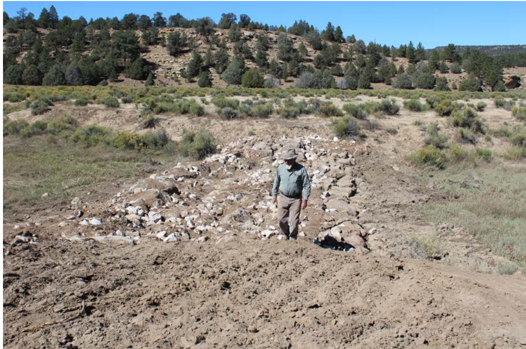
Figure 11. Dam breached and outlet created with heavy equipment to convey flow to center of valley. Larger materials were used on the upstream and downstream edge of the constructed filter dam. Bill Zeedyk (design Contractor) inspects the design and construction results.
