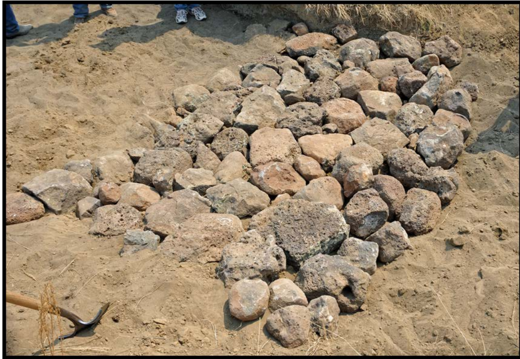
Figure 26. Example of one-rock dam rock work completed in Reach 7 by National Wild Turkey Federation.
