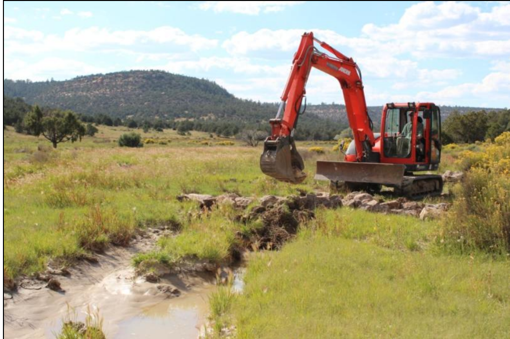
Figures 18a and b (Figure a) An abandoned road was capturing drainage and creating a gully. (Figure b) Newly constructed structure cuts off flow to the ruts and returns flow to valley center.
