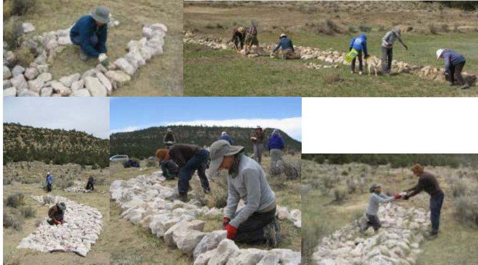
Figure 30. A collage of photos taken of volunteers constructing media lunas on Reach 3 during the April 2014 restoration effort by Albuquerque Wildlife Federation. The photos are from the May 2014 PineCone newsletter article.
