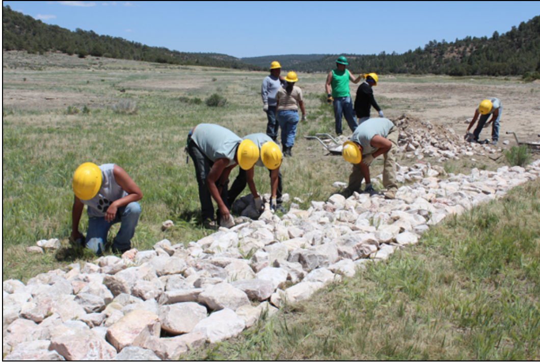
Figure 20. Acoma Pueblo SCC constructing flow dissipation structures.
