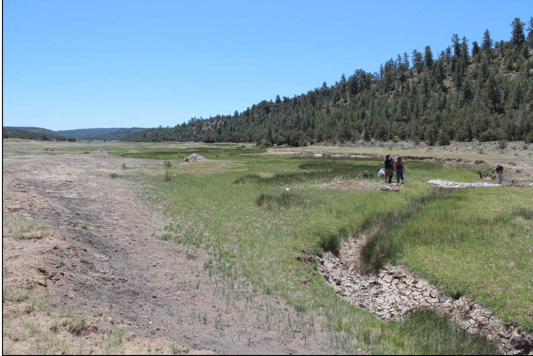
Figure 15. One-Rock Dam grade control structures constructed by volunteers promote the spreading of flow from small incised channels to expand wetland obligate species and groundwater infiltration across the valley floor. In the background are piles of rock staged for hand placement in designed structures.
