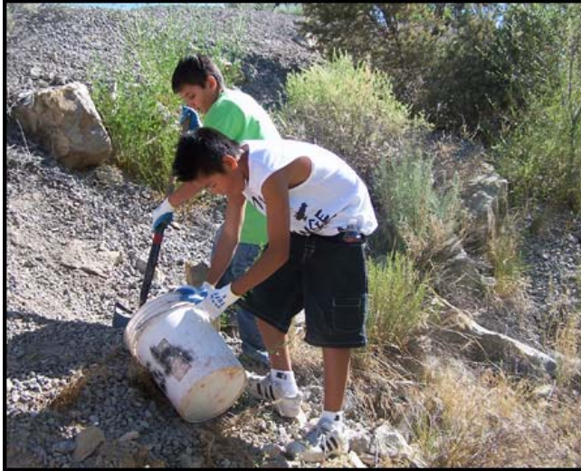
Students collect gravel to help construct one of the restoration structures.
