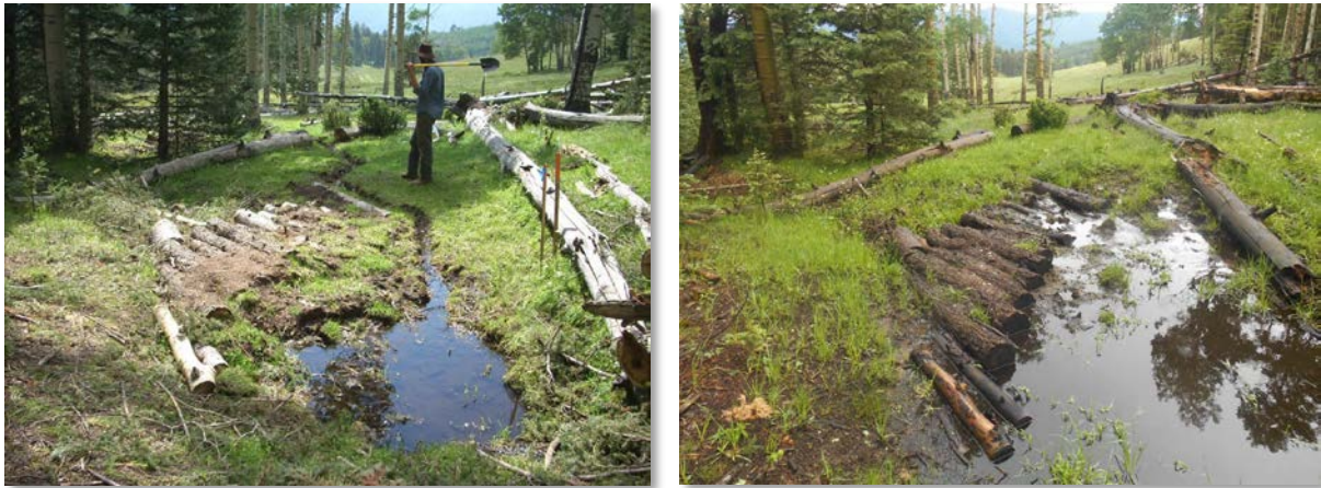
Figure 14. A log mat was installed in at Site 15 in Upper Springwagon Creek to raise the channel and lateral worm ditch was dug to redirect flow to rewet a meadow. Photo taken August 2013 just after installation ( left ). Figure 15. Site 15 in Upper Springwagon Creek two years after log mat and worm ditch Photo August 2013 just after completion ( right ).
