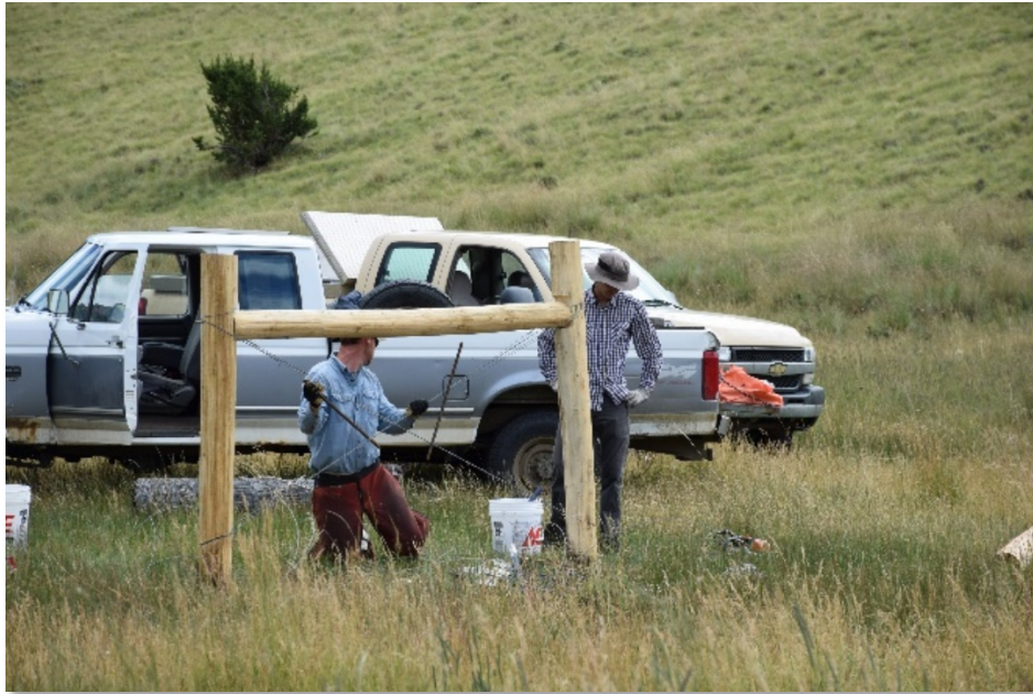
Figure 28. Construction of a livestock exclosure fence around one of the plug and pond structures in a sensitive wetland area in Upper Grassy Creek in August 2016.
