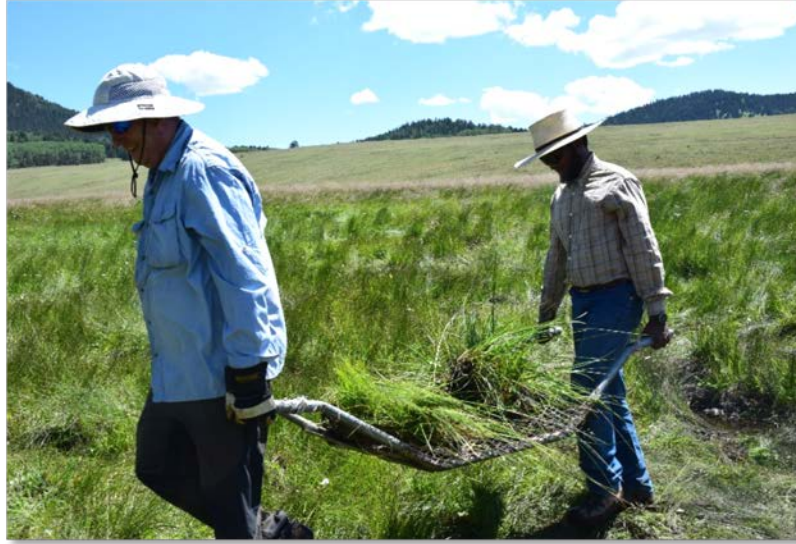
Figure 34. Volunteers carrying sod to use for sod plugs and to fill gaps in step fall structures and Zuni bowls at the August 2014 restoration workshop in Upper Grassy Creek.
