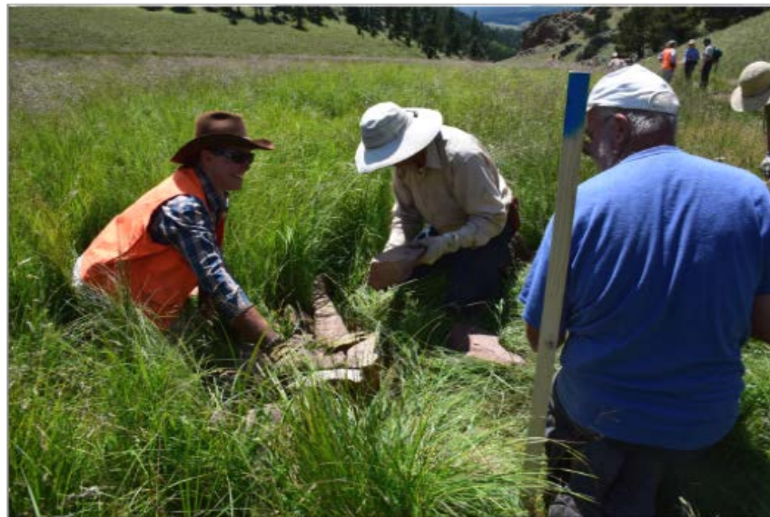
Figure 5. Volunteers constructing small one-rock dams in Upper Grassy Creek.
