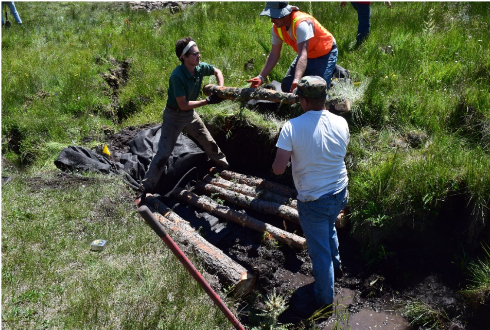
Figure 17. Volunteers building a log step fall structure in Upper Grassy Creek at the August 2014 workshop.
