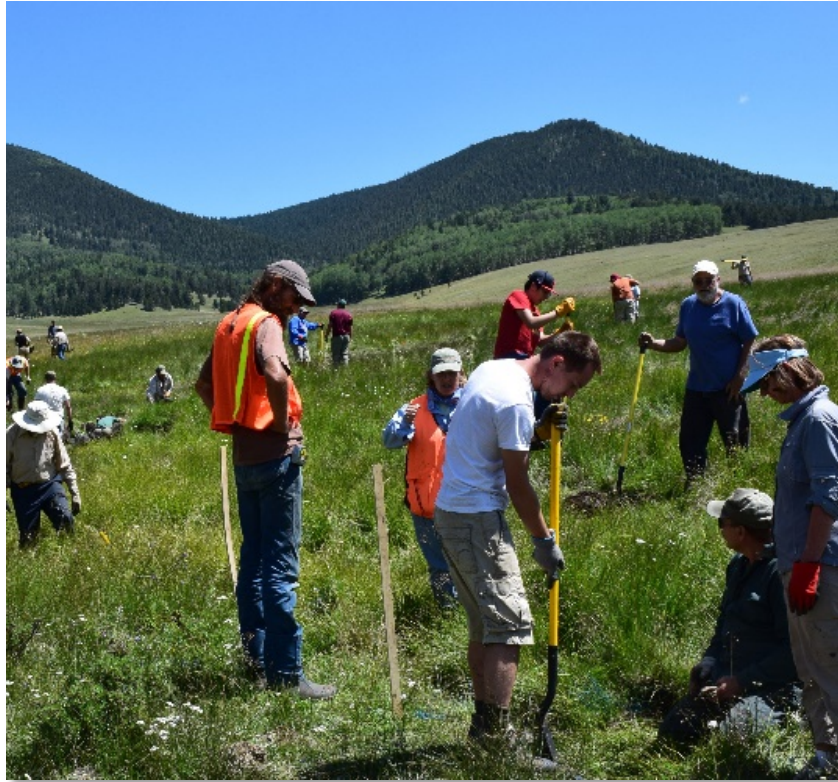
Figure 4. Volunteers digging wetland sod for installing sod plugs into small gullies and for filling gaps in log step fall and Zuni bowl structures in Upper Grassy Creek.
