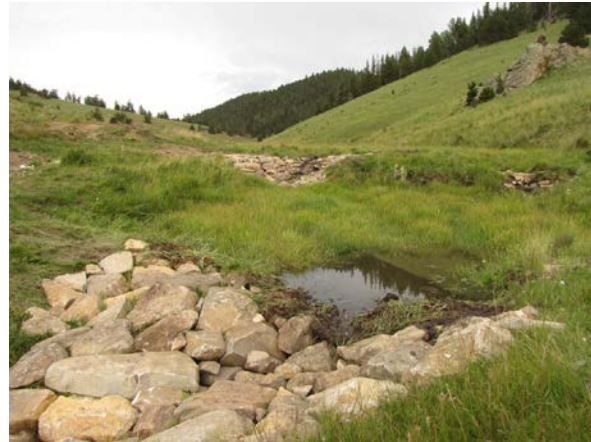
Figure 25. Site 13, Lower Grassy Creek. Series of advancing headcuts, August 2013 (left). Figure 26. Site 13, two years later after stabilization with Zuni bowls built by the subcontractors, August 2015 (right).
