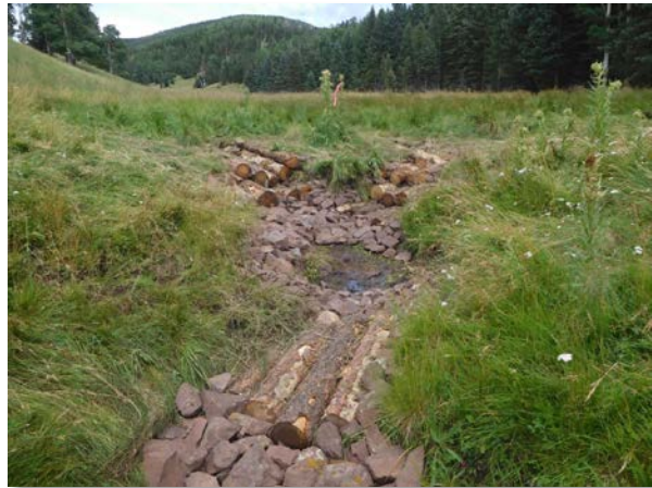
Figure 29. Site 1, Upper Springwagon Creek, shows a migrating headcut, July 2013 (left). Figure 30. Site 1, immediately after installation of a log step fall and rock rundown structure to arrest the headcut in August 2016 (right).
