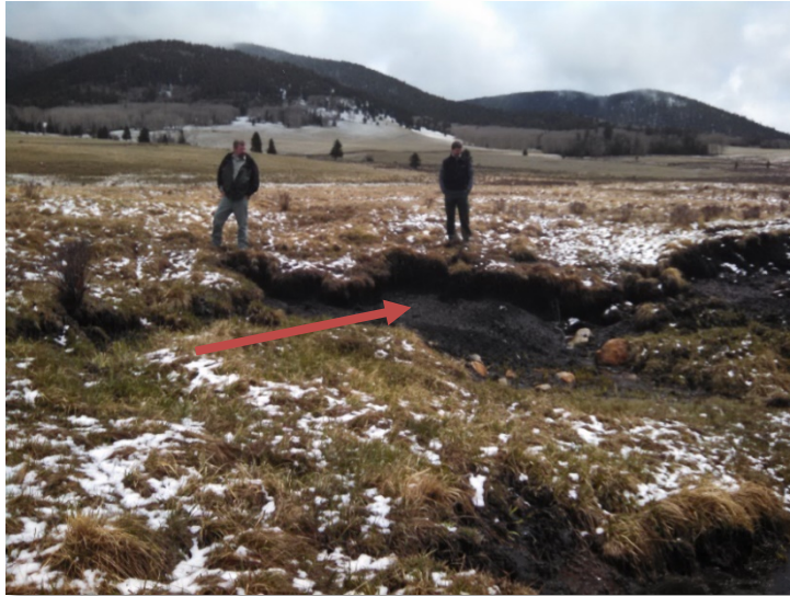
Figure 23. Holman Creek during May 5, 2015 field trip. The red arrow points to a headcut that was draining a five-acre fen. The headcut was stabilized in 2015 by installing a Zuni bowl with funds from Coca Cola Company.
