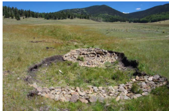
Figure 11. Advancing headcut at Treatment Area Site 17 on Upper Grassy Creek, a tributary to Comanche Creek ( left ). Figure 12. The site was treated with a Zuni bowl and one rock dam to stop headcut advancement ( right ).
