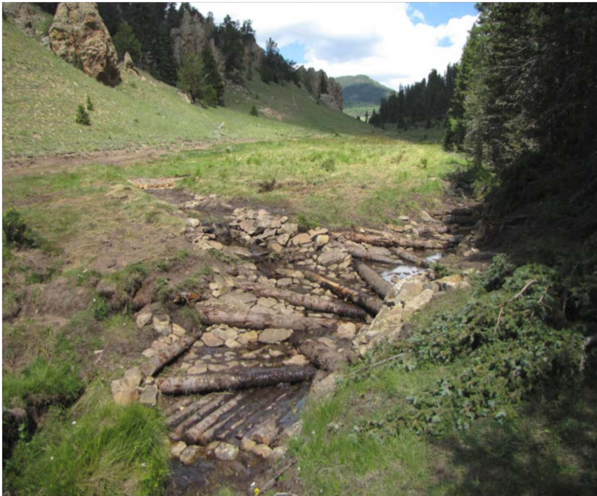
Figure 18. Site 10 in Lower Grassy Creek had a large headcut in a steep section of the channel ( top left ). Figure 19. Subcontractors used machinery to construct a log-rock rundown structure in August
