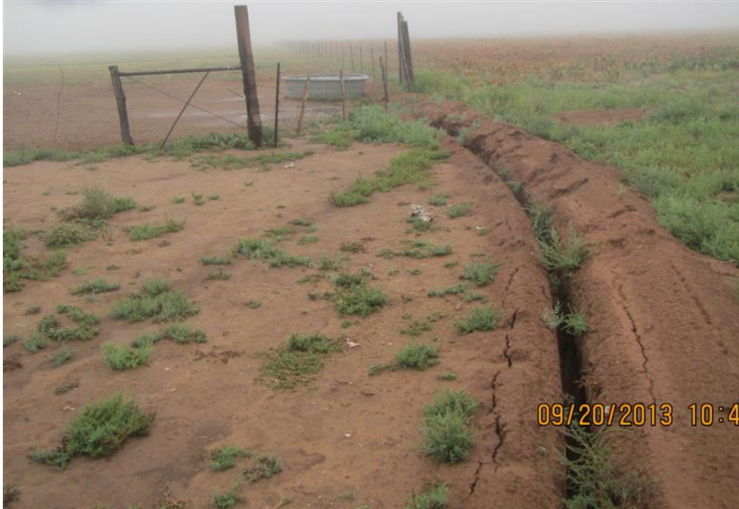
Pipeline installation for upland livestock watering facility at the White playa.
