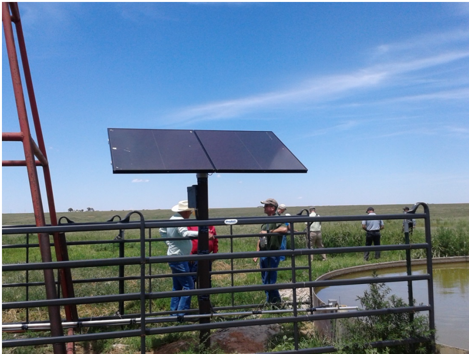
Solar panels with protective fencing for pump to supply upland livestock watering facility at the Tarver playa.
