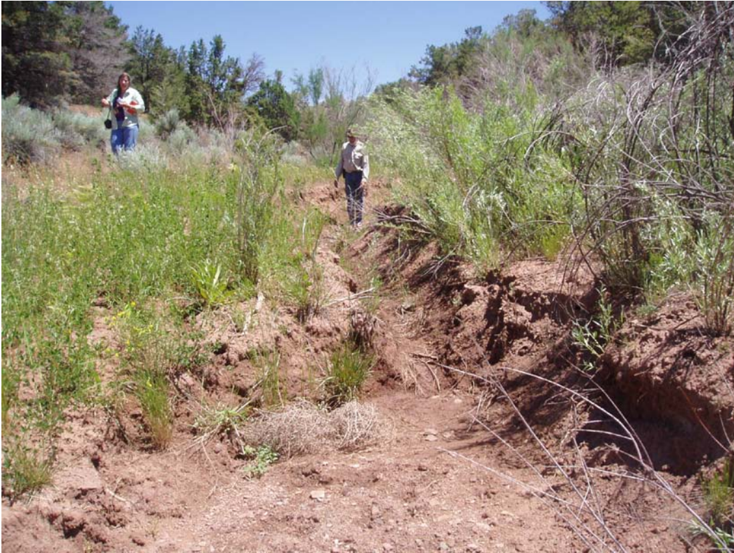
Headcut moving upstream through coyote willow towards Canoncito Arroyo Wetland (2005).
