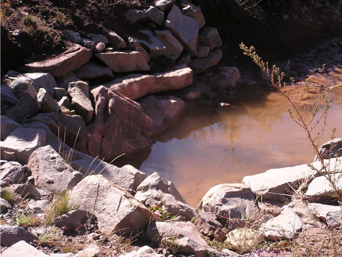
(Above) Rock structures (Zuni Bowl) installed at Canoncito to prevent further headcut. (Below) One rock dam to restore riffle in entrenched reach.
