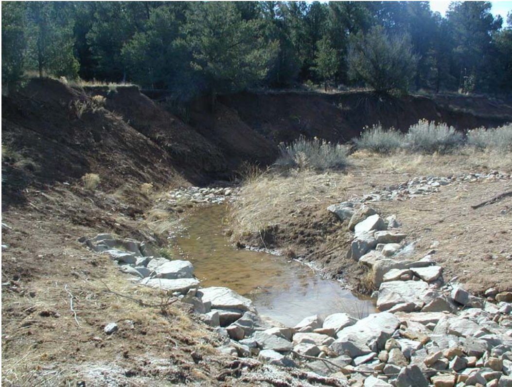
Figure 4. Restoration structures and Canoncito
