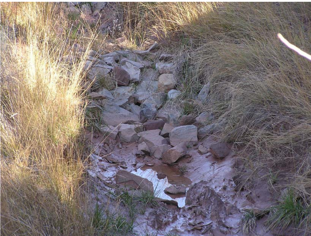
(Above) Rock structures (Zuni Bowl) installed at Canoncito to prevent further headcut. (Below) One rock dam to restore riffle in entrenched reach.
