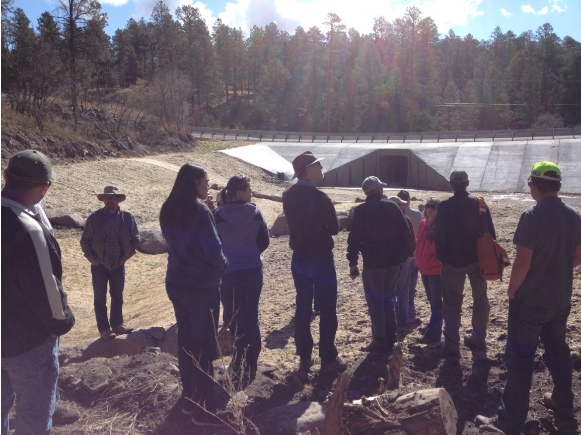
“What’s wrong with this structure?” Workshop field trip site to a poorly designed culvert near Los Alamos in the mountains in a previously burned area serving a fairly large watershed.
