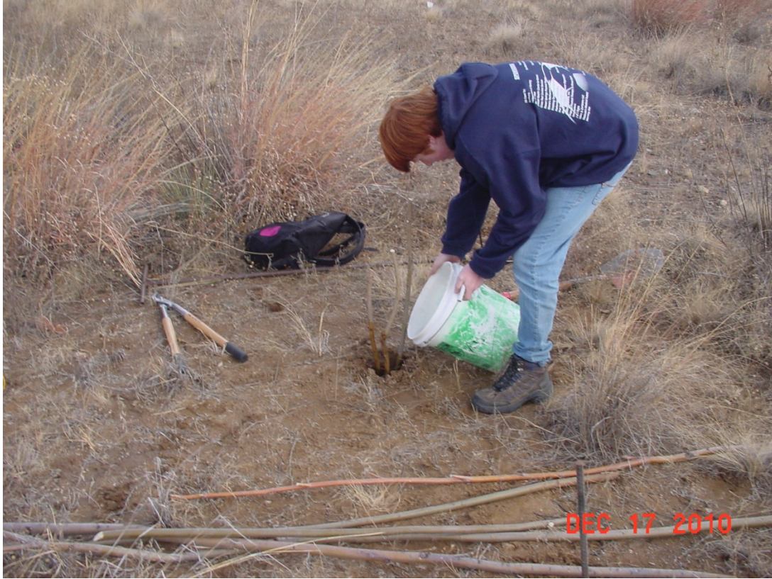
Watering in willow stakes (above) and construction of cross-vane (below)
