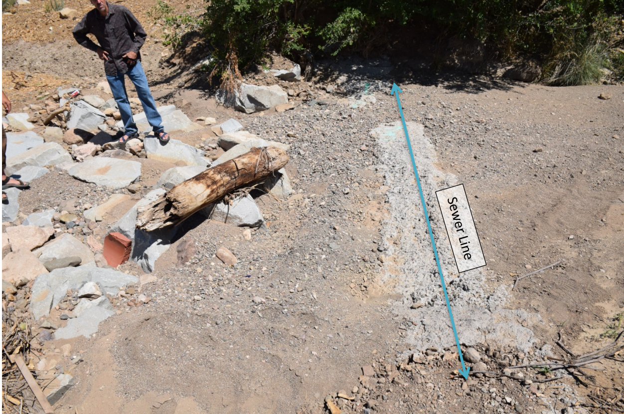
Post flooding sediment deposition. Sewer line now protected from scour by cross-vane.
