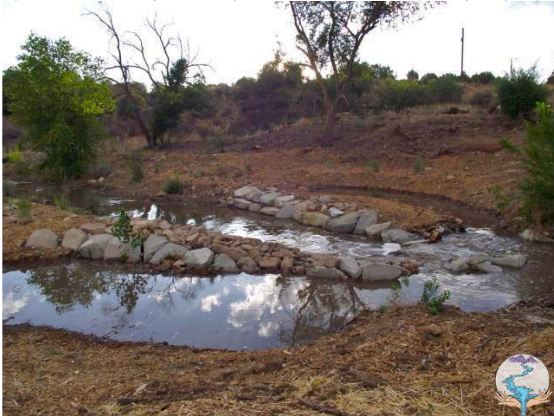
Completed cross vane during a moderate flood event with flood waters spreading onto floodplain.
