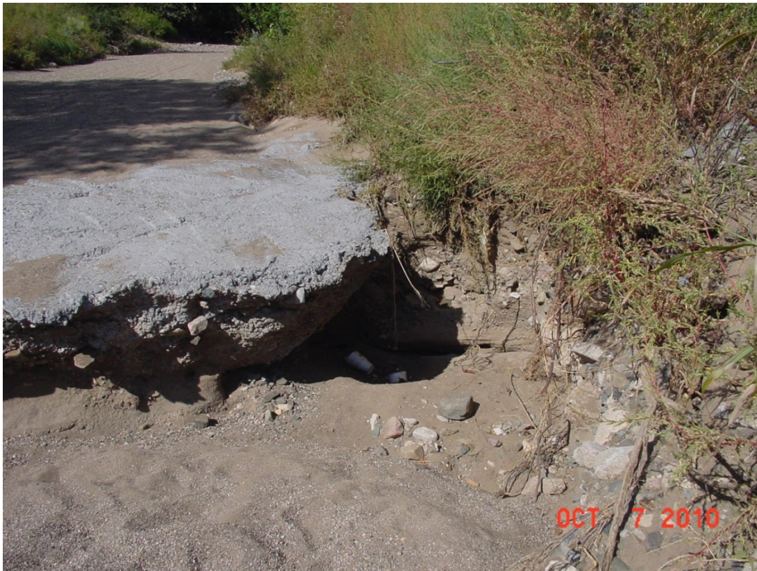
Main sewer line for Silver City crossing San Vicente Creek. Deep scour on the downstream side has compromised the concrete protection.
