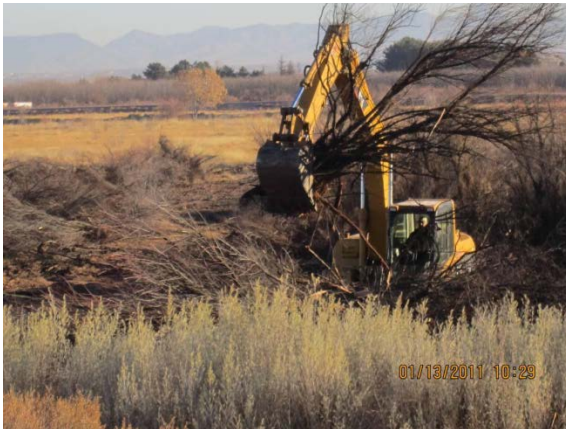
Excavator with “thumb”attachment.
