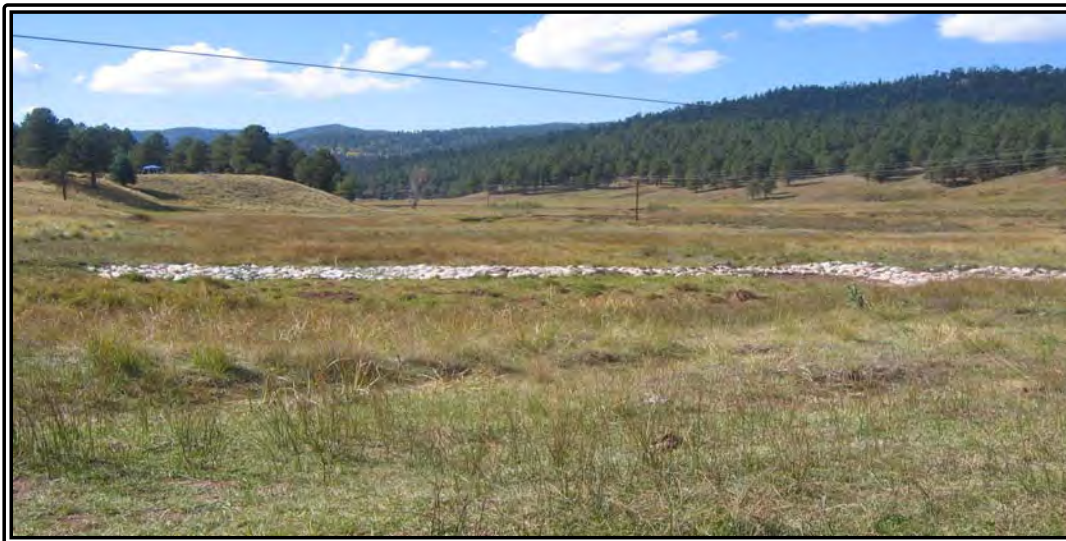
Photo 11. Flow splitter on School Section Canyon
