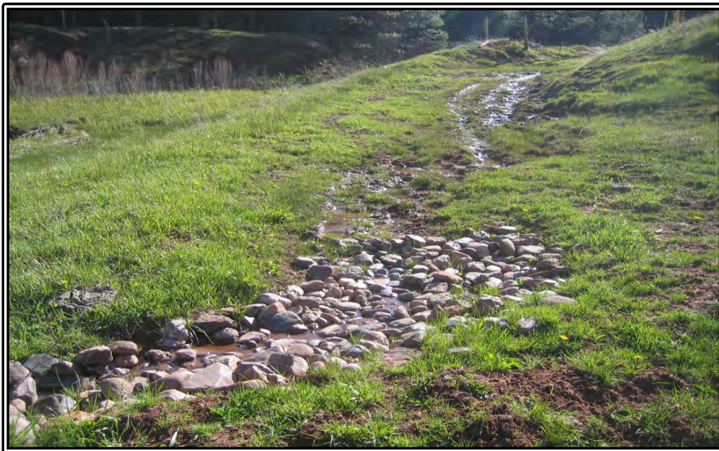
Photo 9. Turkey Canyon springs. One rock dam
