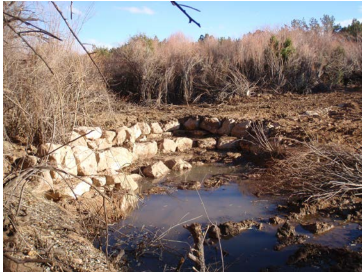
A rock apron is buried below the spring water as part of the Zuni Bowl structure.
