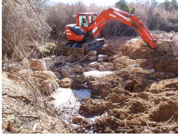
Construction of drop-down structures (Zuni-Bowl) in eroding headcut at San Marcos wetlands
