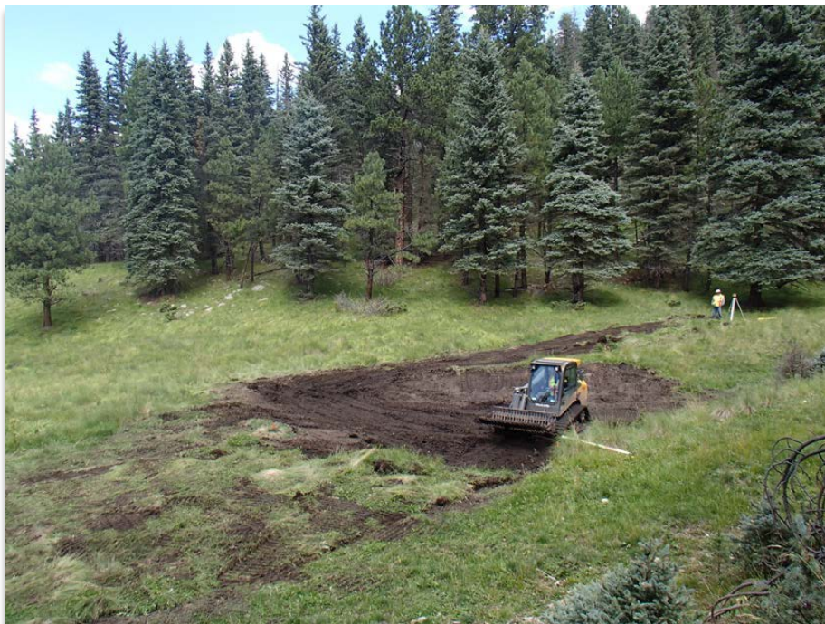
Figure 32. Road work included this machine-built Zuni bowl that collects runoff from Road VC08 (September 2016).
