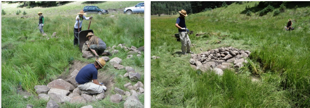
Figure 37. Volunteers carrying boulders to build one-rock dams and Zuni bowls (July 2016).
