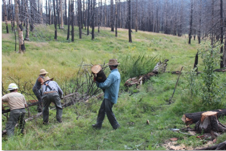
Figure 22. Volunteers stuffing a felled tree into a channel in the burn area at the headwaters of Tributary 1. The tree plugs the channel and causes flow to spill out onto the wetlands (August 2015).
