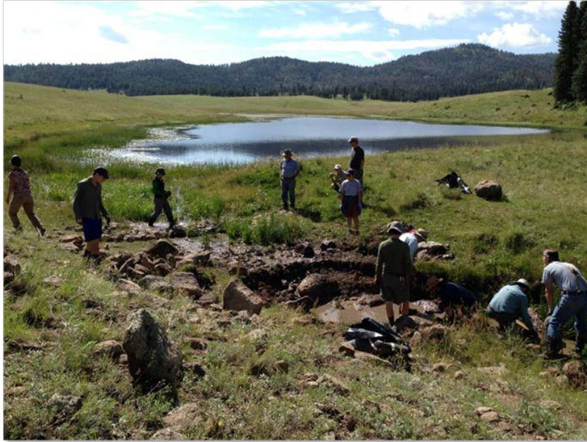
Figure 7. Volunteers constructing a series of zuni bowls and one rock dam to stabilize the spillway of an historic pond at Valle Seco (June 2016).
