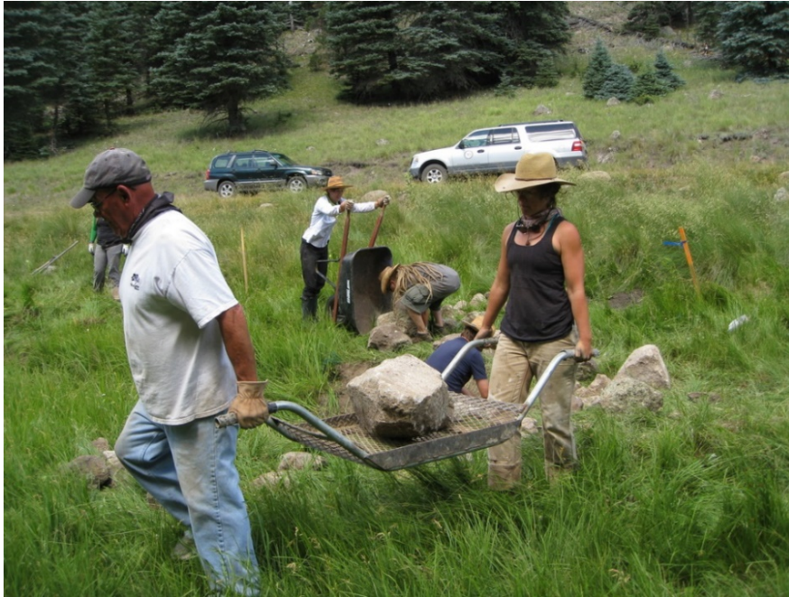
Figure 37. Volunteers carrying boulders to build one-rock dams and Zuni bowls (July 2016).
