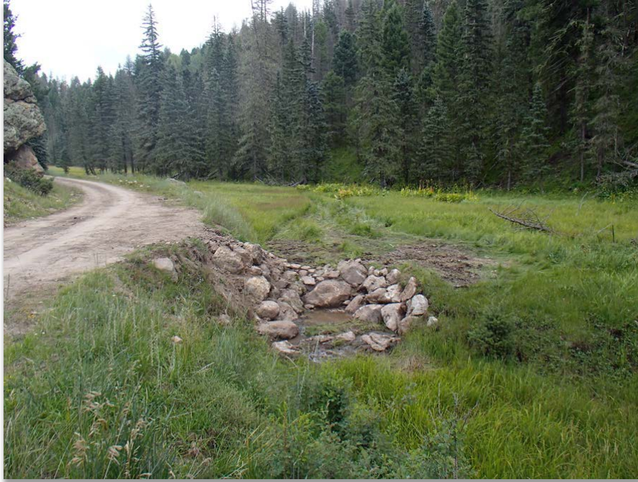
Figure 32. Road work included this machine-built Zuni bowl that collects runoff from Road VC08 (September 2016).
