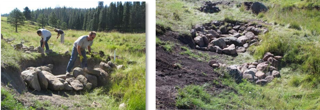
Figure 25. Volunteers building Zuni bowls to prevent headcuts from advancing upstream (August 2015).
