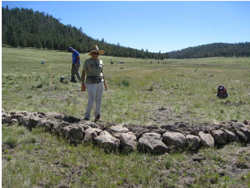
Figure 29. A completed media luna will spread surface water to rewet historic wetlands. Looking upstream in Valle Seco (June 2016).
