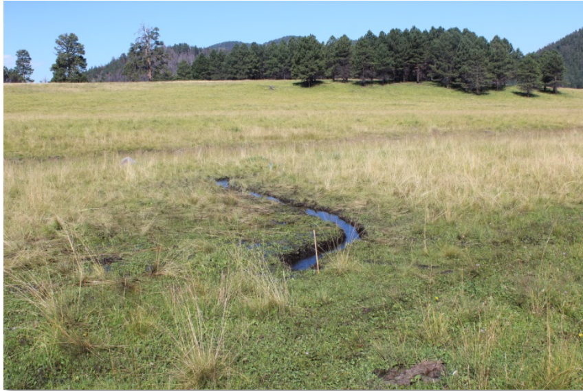
Figure 24. Worm ditch completed by volunteers as it began to spread water across the valley (August 2015).
