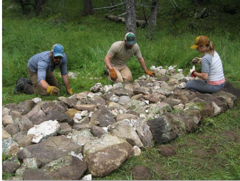
Figure 39. Volunteers building a one rock dam to raise the water table and capture sediment along Sulphur Creek (August 2017).
