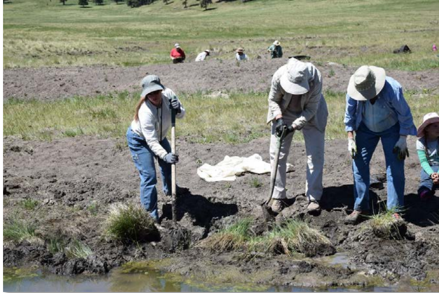
Figure 28. Volunteers transplanting sod to vegetate the perimeter of a plug and pond structure (June 2016).
