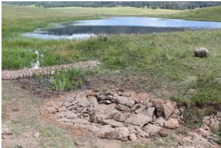
Figure 18. Completed one rock dam and Zuni bowl (center of photo). The Zuni bowl is the same structure shown under construction in Figure 17 (July 2015).
