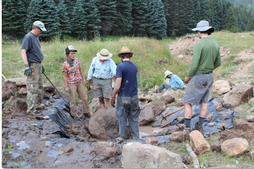
Figure 17. Volunteers considering placement of a large anchor rock in a Zuni bowl. Geotextile fabric was laid under the zuni bowl to help capture sediment (July 2015).
