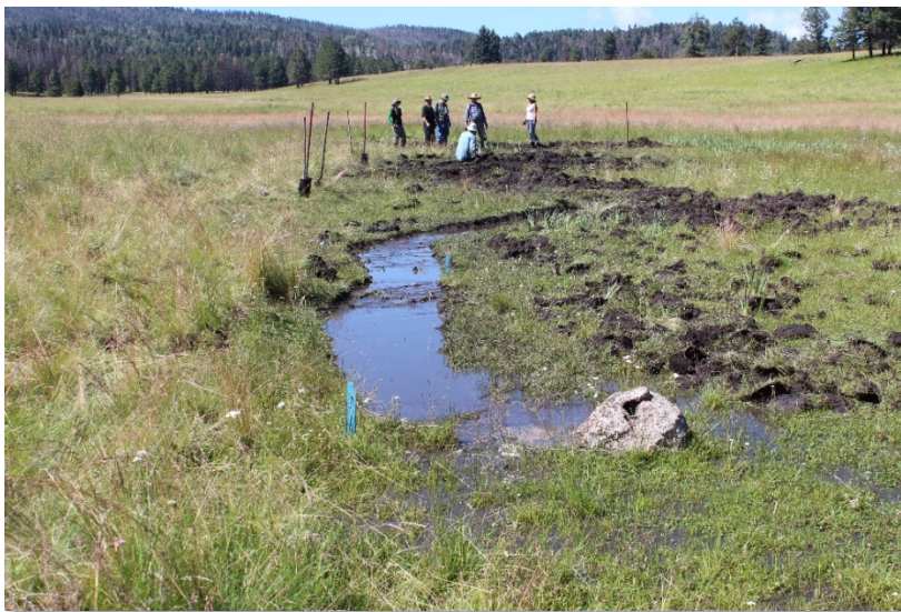
Figure 20. Volunteers completing a worm ditch. This photo is looking upslope and water is spilling out of the worm ditch in the foreground. When working in a wet area, the new flow paths are apparent immediately. (July 2015)
