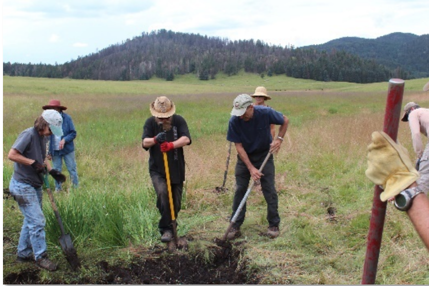
Figure 19. Volunteers digging a worm ditch to re-route water in Valle Seco (July 2015).
