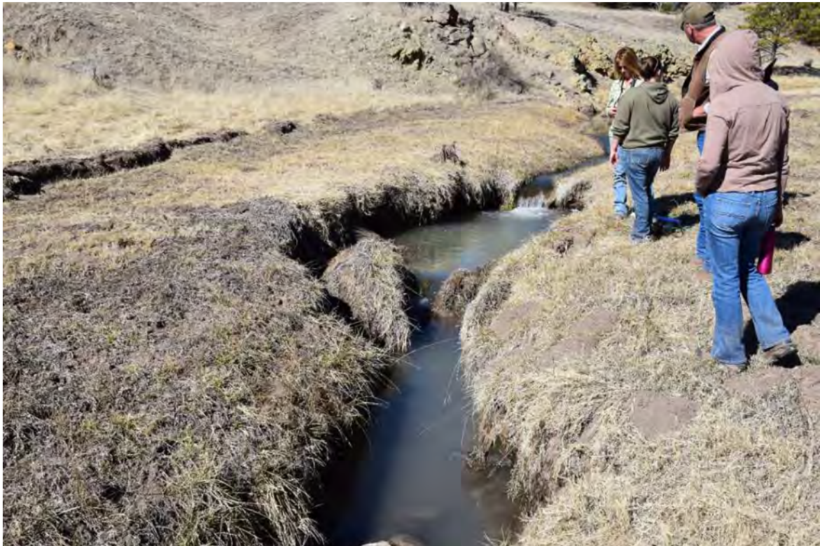
Figure 19. Streambank instability in Centerfire Creek
