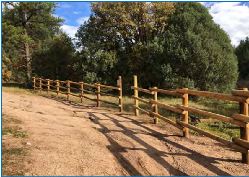
Figure 2. View of the vehicle exclusion fence from along Forest Road #376.
