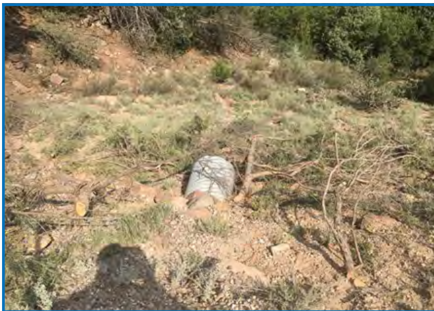
Figure 1. Outlet View of the existing culvert at Joaquin Canyon crossing with Forest Road #376. During the BAER Assessment in August 2018.
