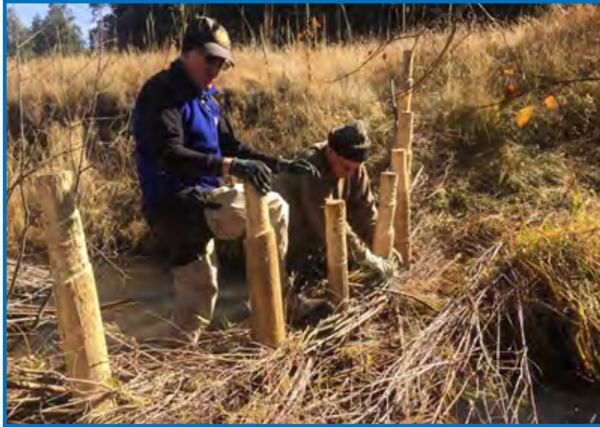
Figure 3. Constructing Beaver Dam Analogs in the Rio Cebolla.
