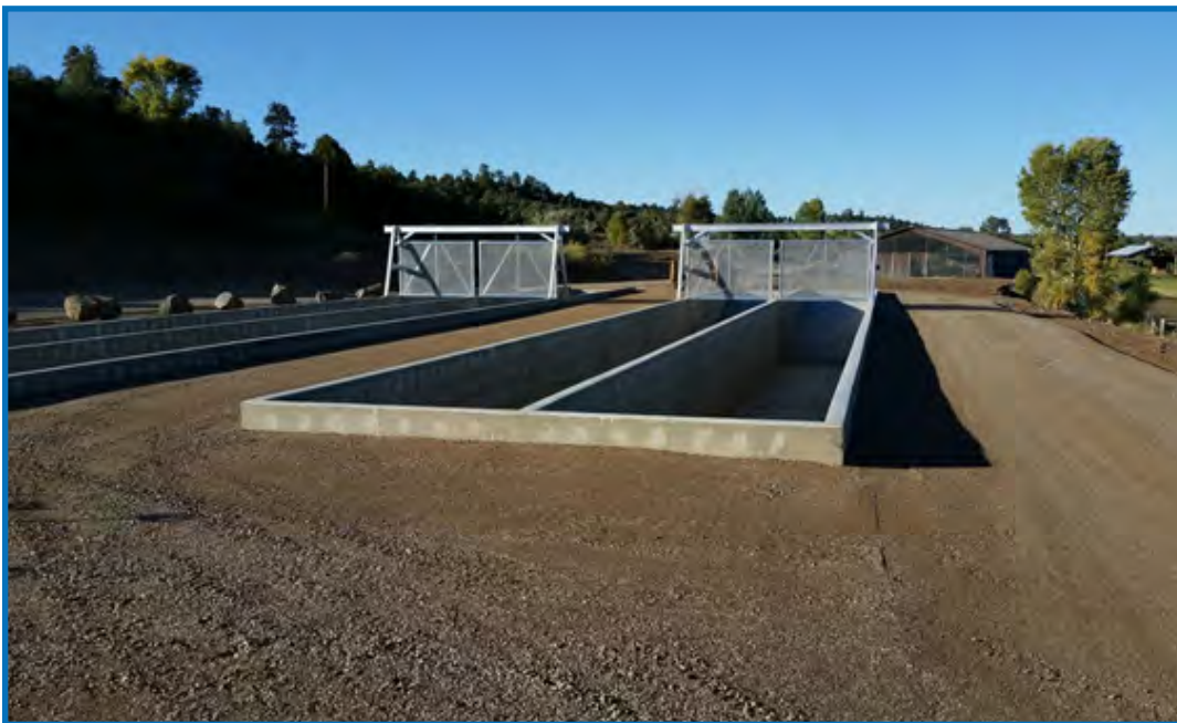
New particulate retention vaults installed at the Los Ojos Fish Hatchery.
