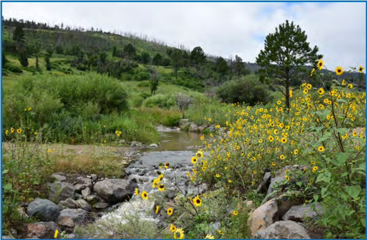
Segerstrom Creek upstream of Lake Maloya. An example cross-vane is visible in the foreground, and a stabilized bank is visible in the background.
