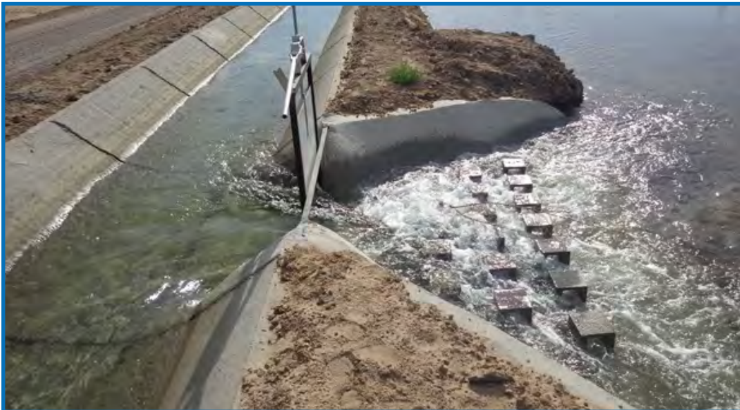
Top picture shows cover crops planted through the NWQI. Bottom picture shows concrete ditch with a structure for water control also implemented through NWQI.
