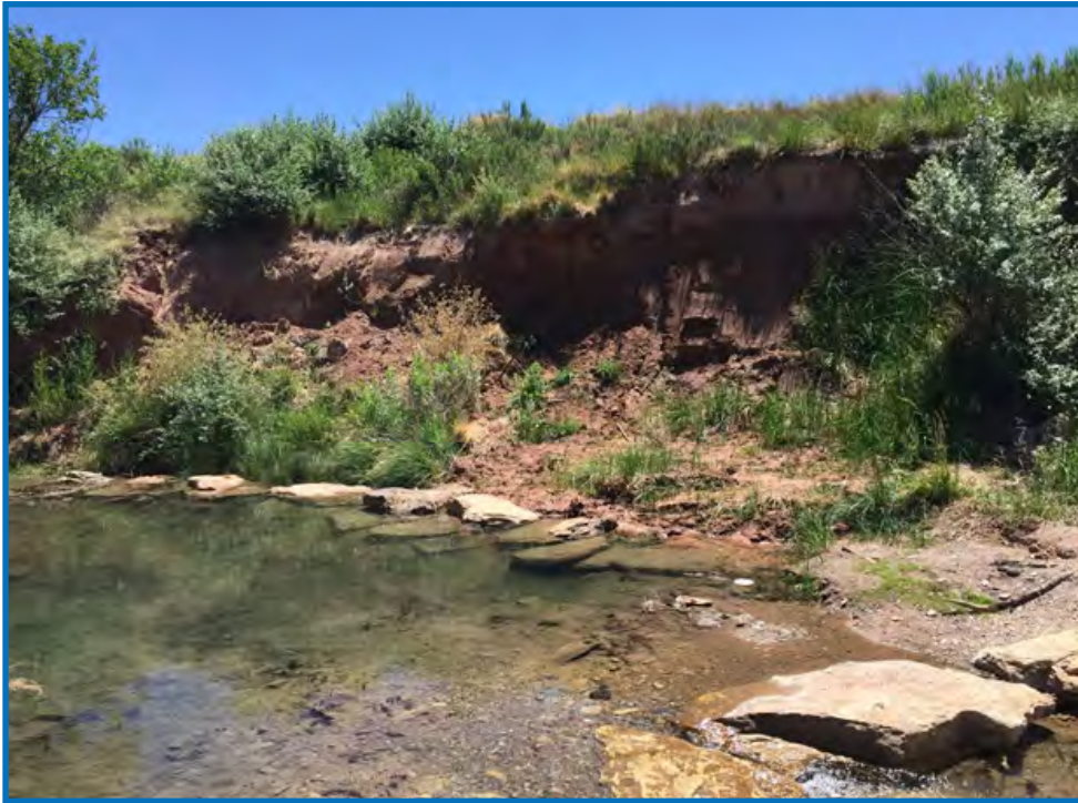
El Rito Creek, near Santa Rosa New Mexico. Example of a bank stabilization (toe rock) structure tied into a cross vane. Note wetland vegetation associated with a spring at left of photo and riparian woody vegetation colonizing streambank behind structure on the left.
