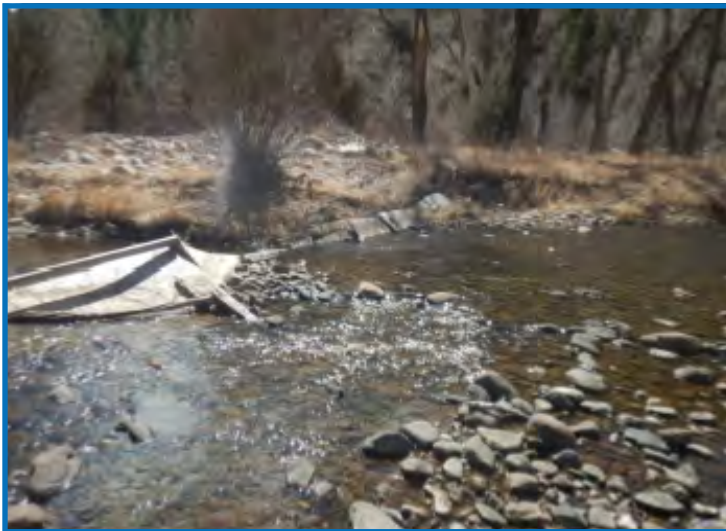
Stream Channel Enhancement - Pre-treatment.
