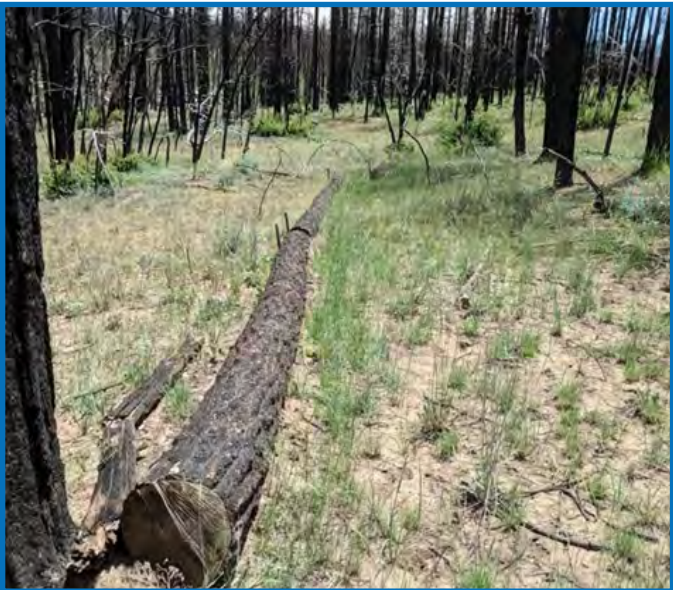
Contour tree felling where sediment was collected and range grasses established.
