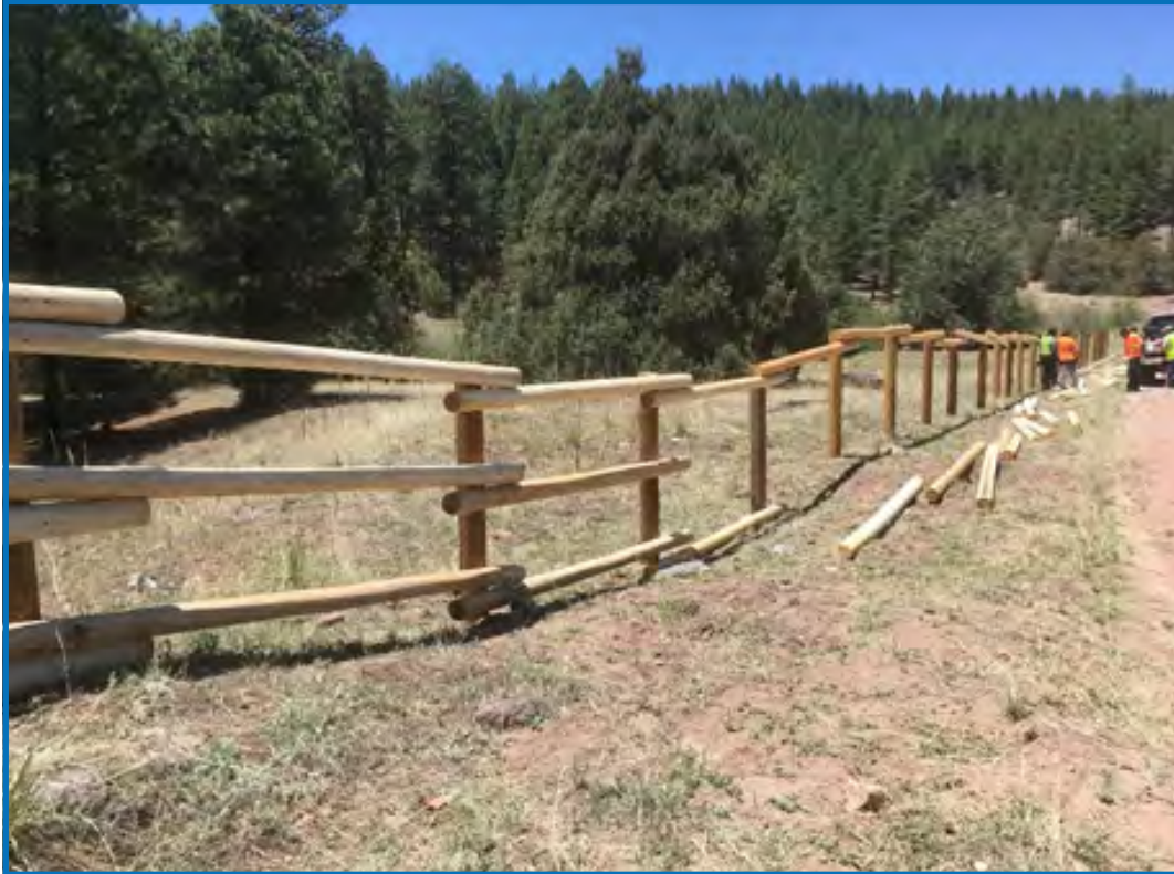
Fencing is installed along critical habitat and wetlands in the Jemez Mountains. The fence will prevent off-road vehicles and cows from impacting the riparian area.
