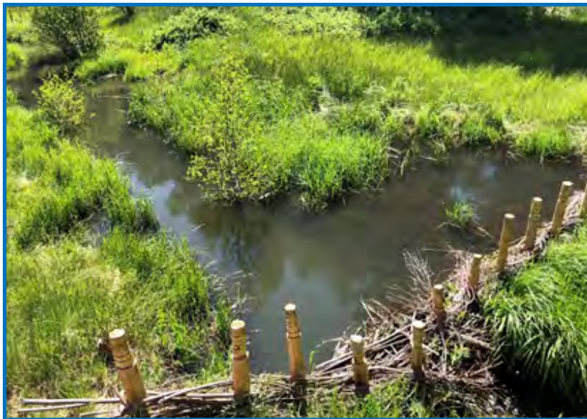
Figure 4. Completed and functioning Beaver Dam Analog in the Rio Cebolla several months after installation.
