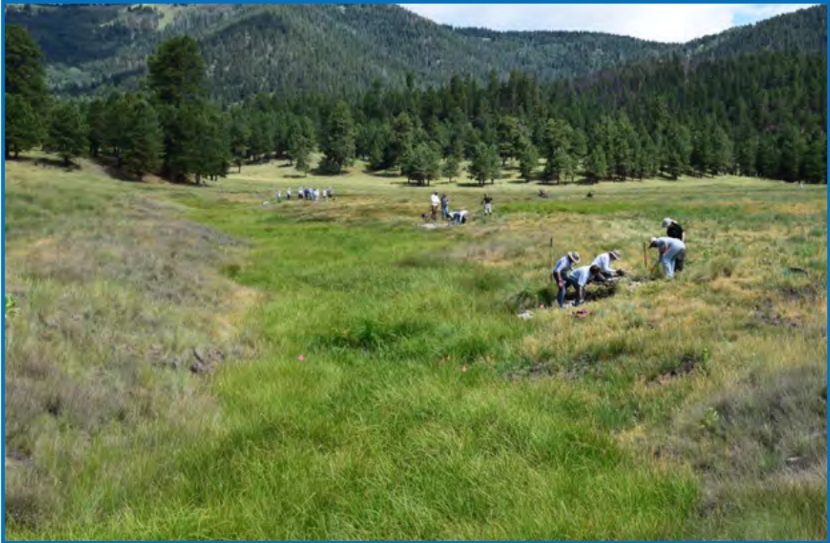
La Garita Creek, a tributary to San Antonio Creek included in this project. Volunteers building rock structures to spread water and arrest erosion.
