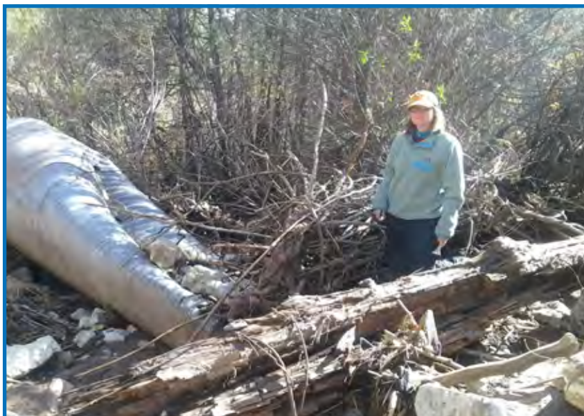
Figure 2. View below culvert outlet of debris and failed section of pipe that blew out.
