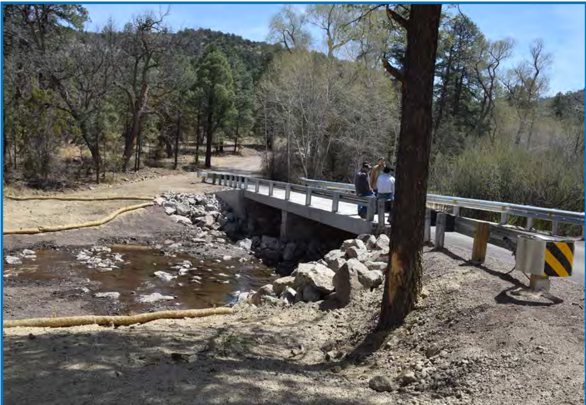
USACE, USFS, NMED and contractor tour recently completed project of Forest Road 150 bridge over Black Canyon Creek in the Gila National Forest. April 2018.
