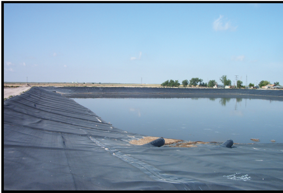
Synthetically-lined Dairy Wastewater Lagoon
