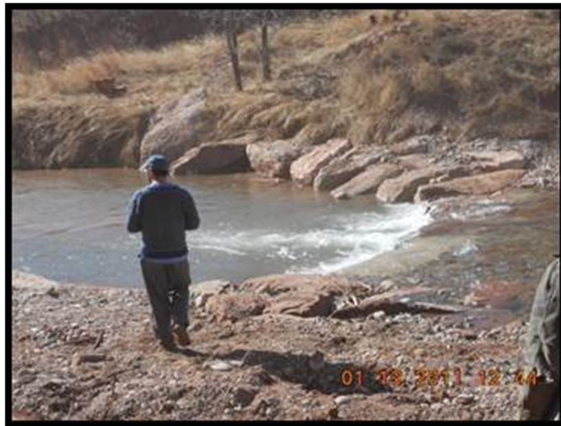
Pecos River Restoration at El Valle: This cross vane on the upper Pecos River was constructed with heavy equipment to control the grade of the river bed, create habitat, and improve aeration.
