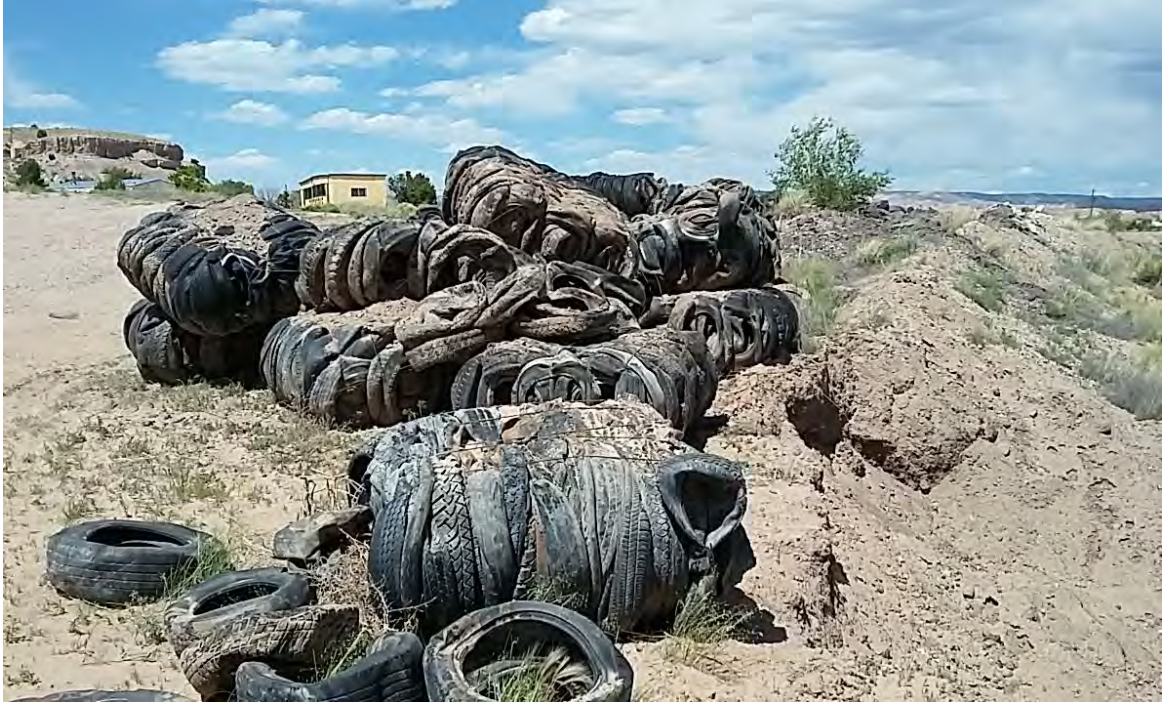
Figure 3: These tire bales were part of a failed streambank stabilization attempt. The tire bales were carried downstream during a flood event, risking downstream culverts and property. The U.S. Army Corps of Engineers Albuquerque District prohibits the use of tires as fill in all waters of the United States and required these bales to be retrieved and removed. Photo by Alan Klatt, May 25, 2017.
