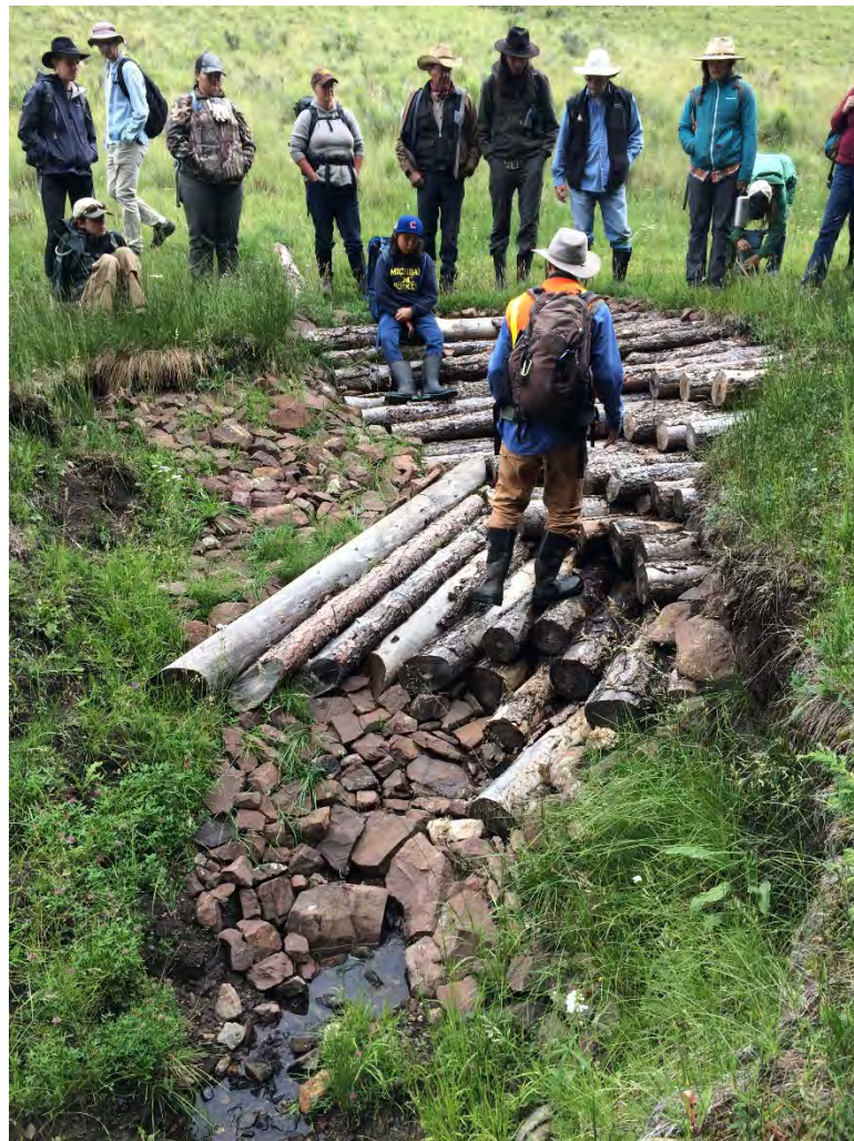
Figure 4: Quivira Coalition workshop participants learn how a log run-down was built to stop a head cut. This head cut had advanced to the lower end of a slope wetland on Springwagon Creek, and further cutting would have drained the wetland and delivered a large amount of sediment to Comanche Creek. (Photograph August 2017 by Abe Franklin).
