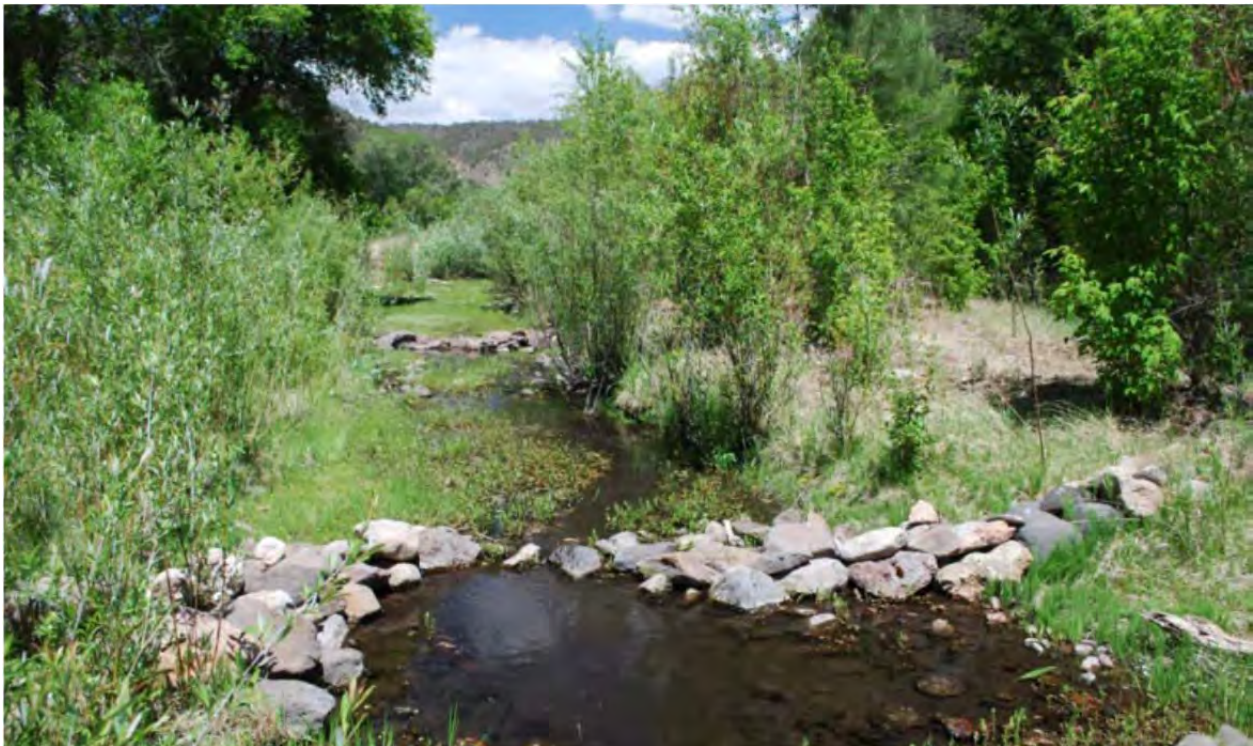
Two of the hand constructed rock weirs in Black Canyon that focus streamflow to encourage scour pool development, enhance fine sediment deposition and riparian vegetation recruitment.
