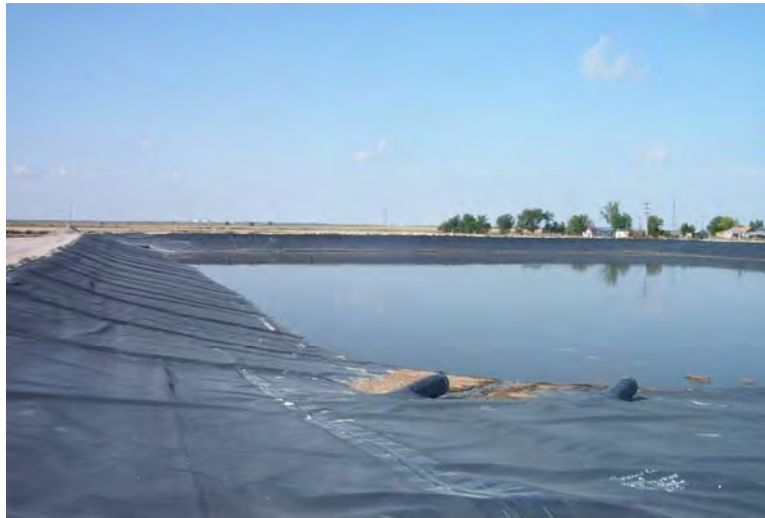
Synthetically-lined Dairy Wastewater Lagoon
