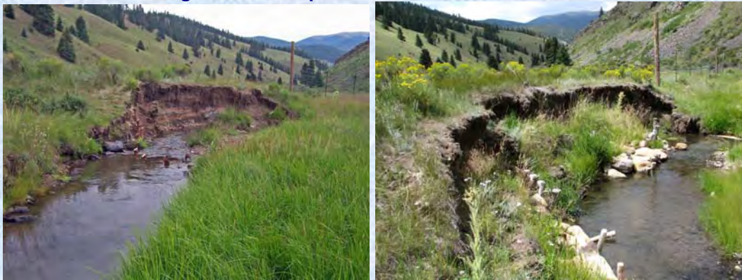
A cut bank on Comanche Creek, before and after treatment.
