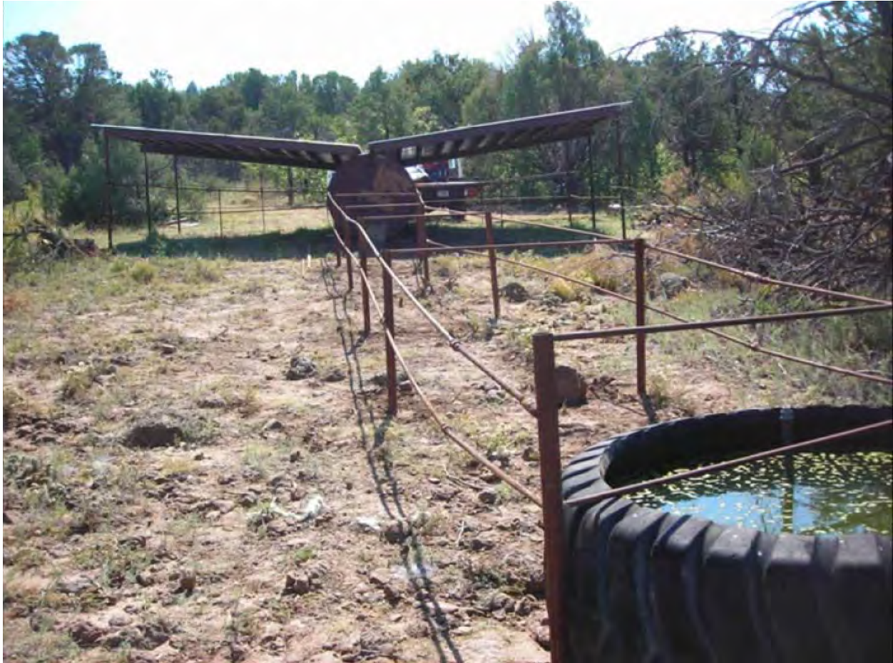
Figure 2: The Cerro Pelon trick tank, constructed on the Polvadera Grazing Allotment in the Española Ranger District, provides an upland water source in a non-riparian pasture, to reduce grazing pressure along Polvadera Creek (Photo by Santa Fe National Forest, Espanola Ranger District staff, summer 2012).
