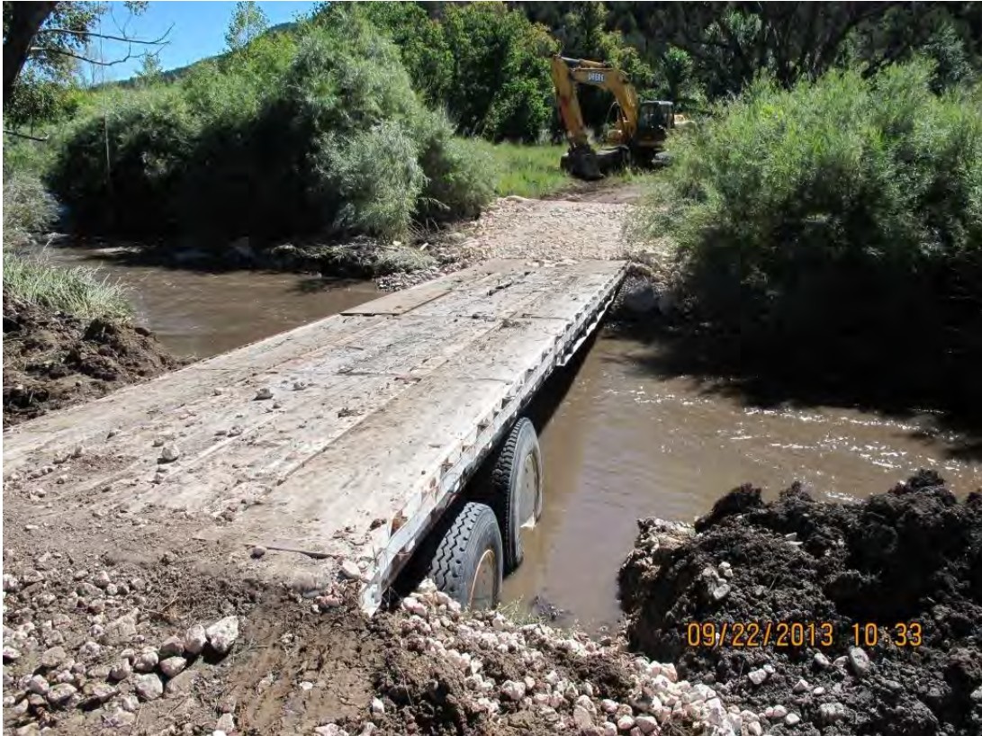
Figure 3: An unauthorized bridge over the Rio Bonito. The BLM, NMED, United States Army Corp of Engineers, and nearby landowners cooperated to remove the bridge, using the authorities of Sections 404 and 401 of the CWA. Photo by Mike McGee, September 22 2013.
