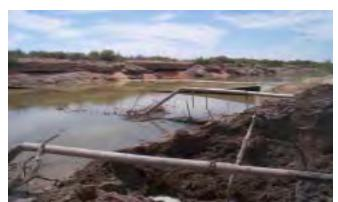
Looking downstream at the Pecos River near the New Mexico-Texas border. Black floating silt fence appears immediately downstream of the pipelines, and two closelyspaced white absorbent booms are deployed downstream of the silt fence. Photo by Mary Jo Rugwell, U.S. Bureau of Land Management
