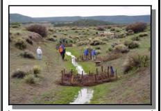
Figure 1: Looking upstream on Largo Creek, a deflector bracketed by wicker weirs will promote development of a meander.
