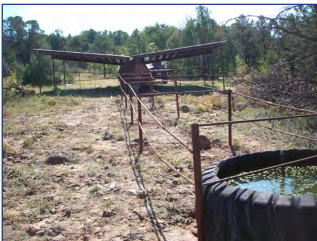
Completed trick tank
