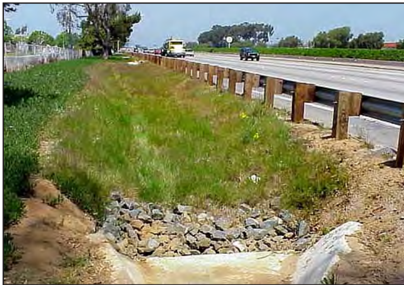
Example of a vegetated swale. Photo courtesy of Caltrans.
