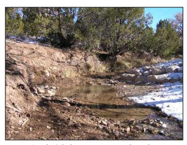
Restoration of deep downcut gully and back-eddy area at Van Driessche/Bladergroen property boundary – (view upstream). Note baffle installation on right and restoration of floodplain. Photos courtesy of R. Bandeen
