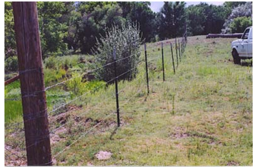
Area after installation of fence on Estrada's place
