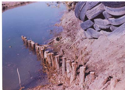
Installed 30' vane structure for erosion control
