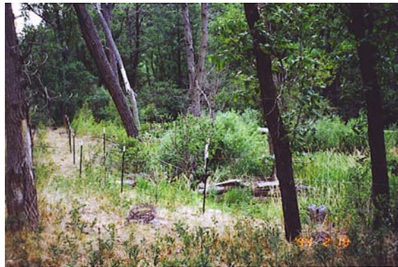
Meyer's fencing project
