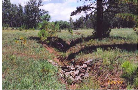
Rock & Brush dams to prevent further erosion
