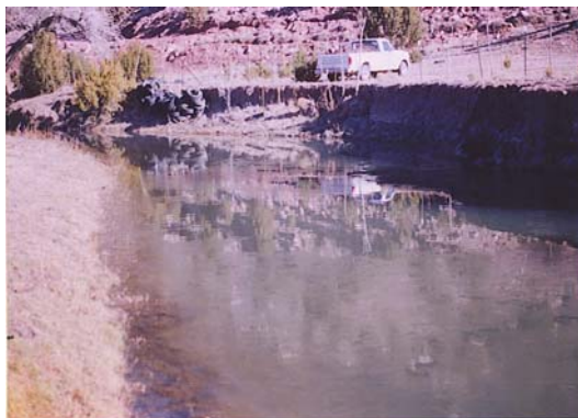
Eroding streambank at Damian Lujan Sr.'s
