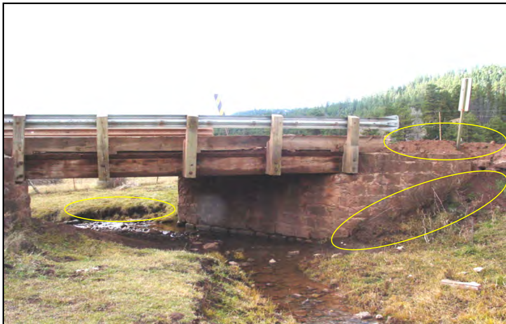
Figure 5. Road maintenance spoils in the Rito Peñas Negras
