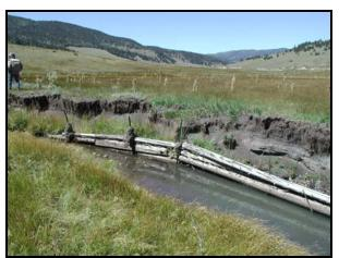
Figure 5 Revetment Structure in Comanche Creek built in the late 1980s
