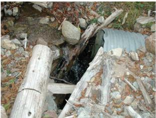
Figure 12 Culvert Opening Almost Plugged
