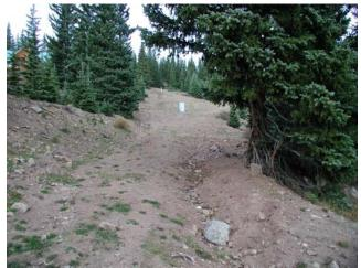
Figure 13 Roads and Ski Runs Have Altered Drainage
