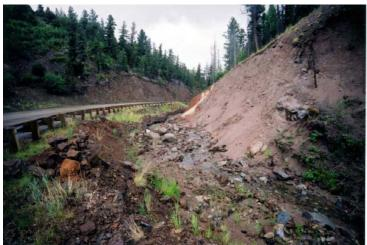
Figure 14 Bank Erosion Along NM 196
