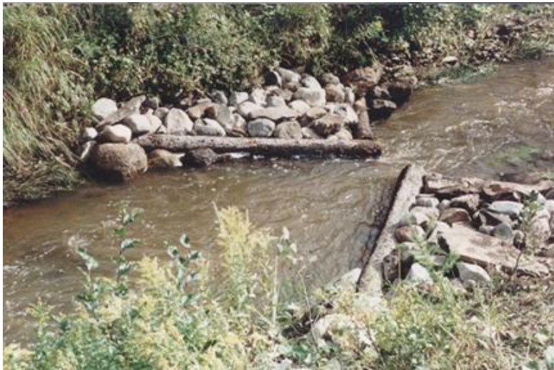
Figure 35: Log deflectors from both banks Image from afterwildfirenm.org
