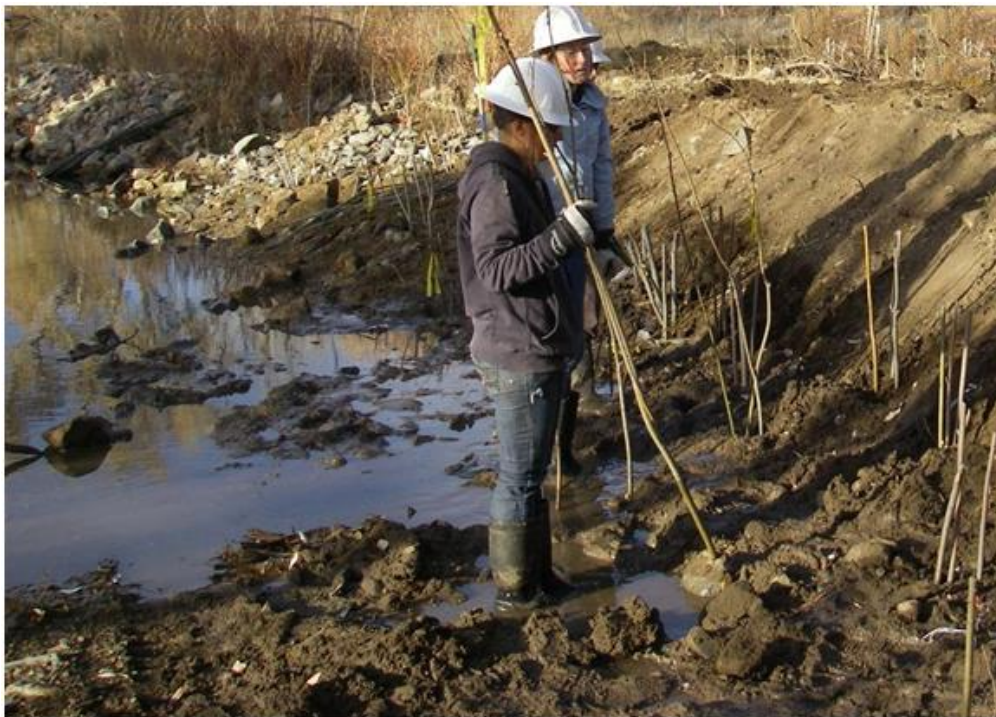
Figure 26: Willow pole plantings at stream bank as part of stream/habitat restoration
