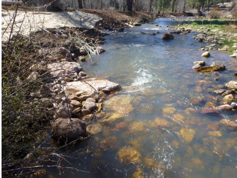
Figure 31: Rock Barb extending from left side into the base flow channel
