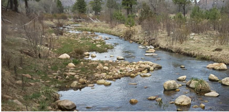
Figure 34: Low deflector built at Canyon Creek, Az.
