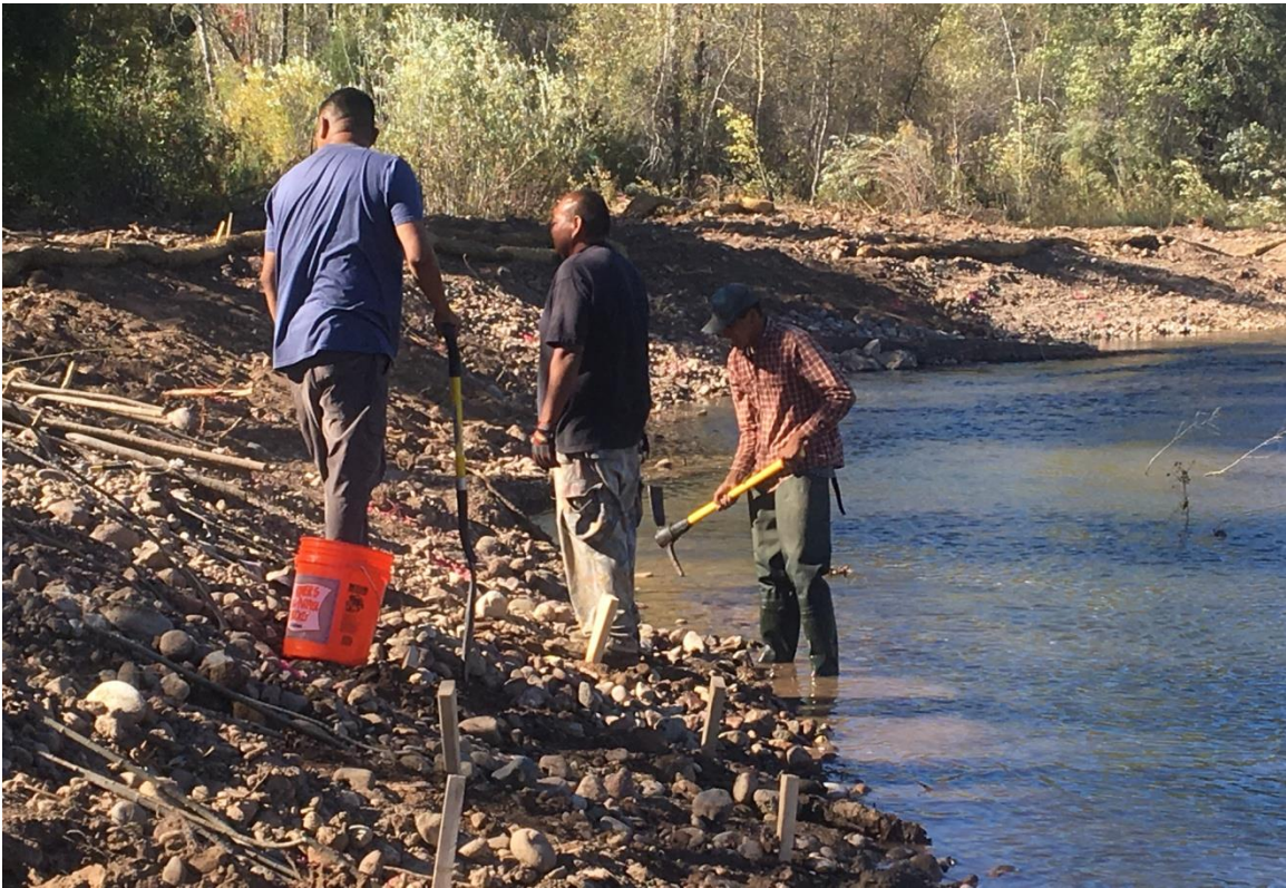
Figure 27: Willow bundles being installed on a river bank
