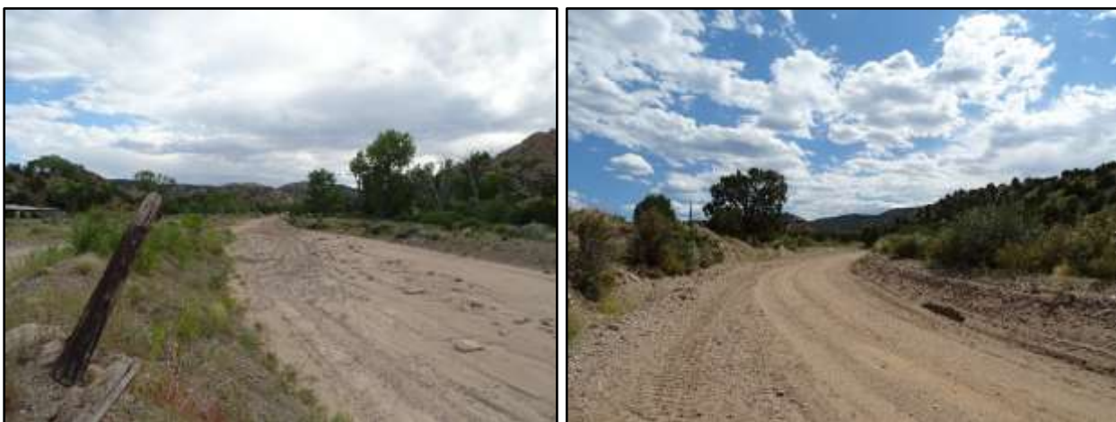
Figures 3.8 (left) and 3.9 (right). Examples of the use of arroyo bottoms as dirt roads and driveways, which constitutes a serious cause and source of erosion and sediment transport.
