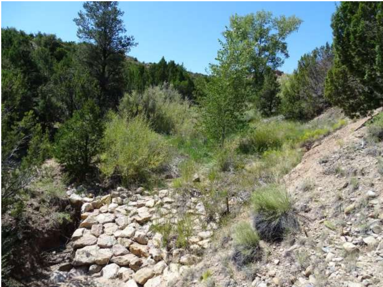
Figure 5.3. Example of a perched wetland on BLM land that was stabilized in 2013 and that retains thousands of tons of sediment in a small watershed on BLM and State Trust Land in the Cañadita del Agua in Cañoncito.
