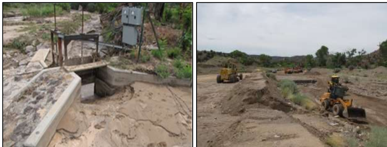
Figures 4.3 (left) and 4.4 (right). Periodic high flow events also cause sediment transport that clogs head gates and acequias (left) and leads to high costs of excavating essential channels and culverts (right).
