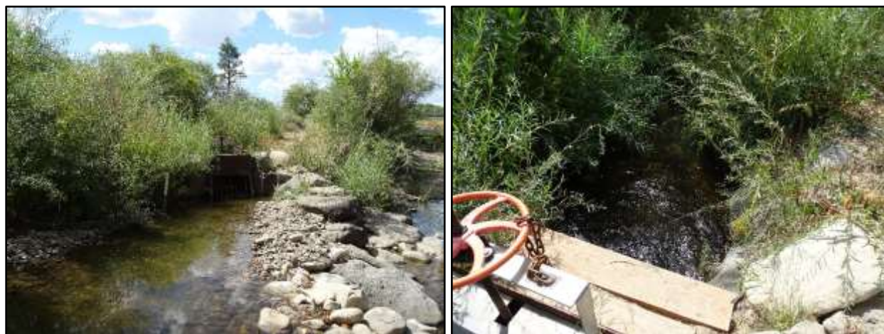
Figure 3.5 (left). Contemporary head gate inlet of the Acequia de la Plaza, one of the first acequias of Dixon. Figure 3.6 (right). Close up view of water flowing from head gate into the acequia system.
