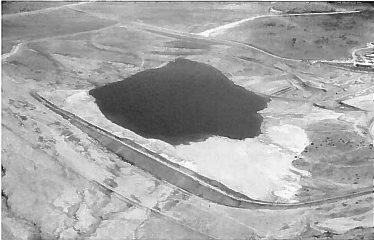
Figure 4. L-Bar Uranium Mill Tailings Impoundment, circa late 1970s.
