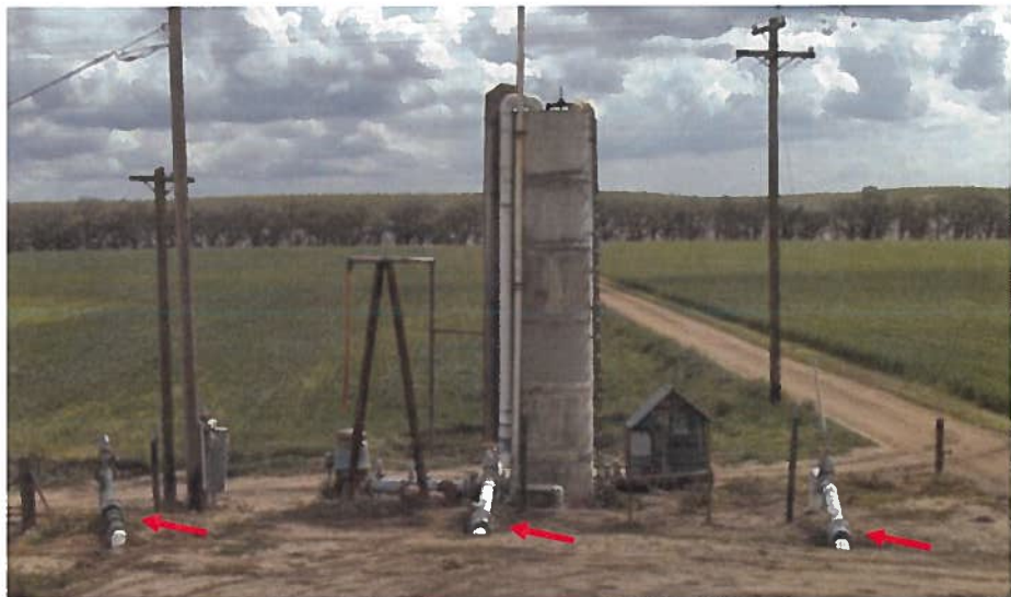
In this installation, separate metering runs allow lagoon water to be accurately applied on three locations simultaneously. A kiosk provides a lit, sheltered location to post target flow rates and record data.
