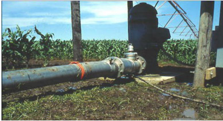
Chemigation check valve next to the well. Note the rubber hose connected to the low pressure drain directs leaking water away from the well.
