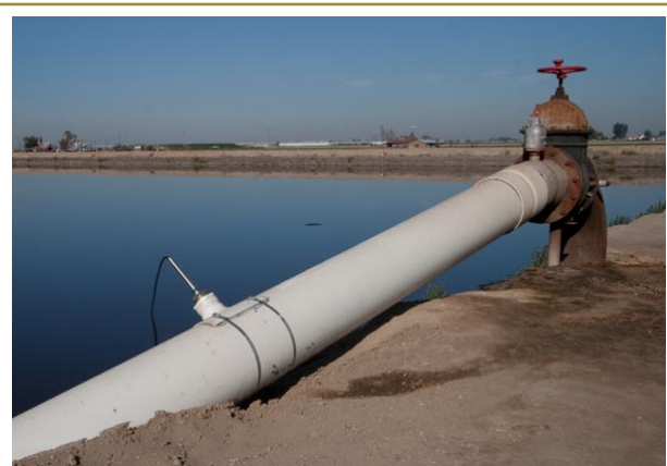
This probe style meter sensor is screwed into a threaded nipple mounted on a PVC saddle. The rise in the pipe beyond the meter assures that the pipe is full.
