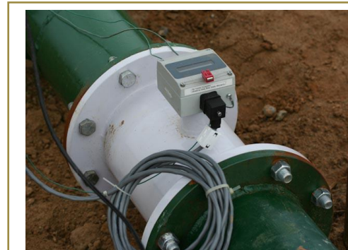
This photo shows an electromagnetic meter that replaces a section of pipe. The terms “spool type,” “tube style” and “full bore” are used interchangeably for this type of meter.
