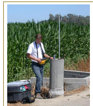
A hand held meter mounted on a rod works well for measuring flow velocity at a single point in time. The velocity should be measured at several points across the transect of the pipe if using an electromagnetic or propeller meter.
