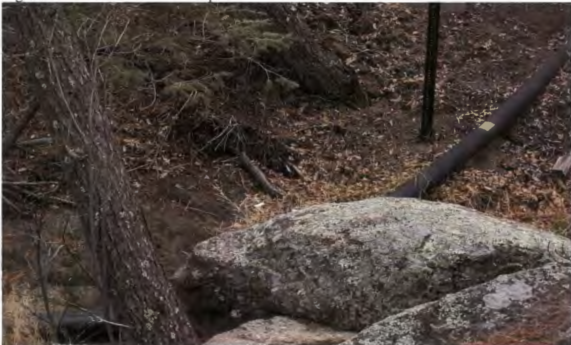
Figure 30. Effluent Extension Pipe.
