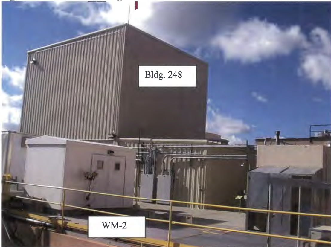
Figure 22. WM-2 and Building 248.
