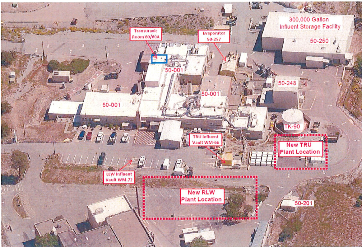
Figure 1. Aerial View Radioactive Liquid Waste Treatment Facility
