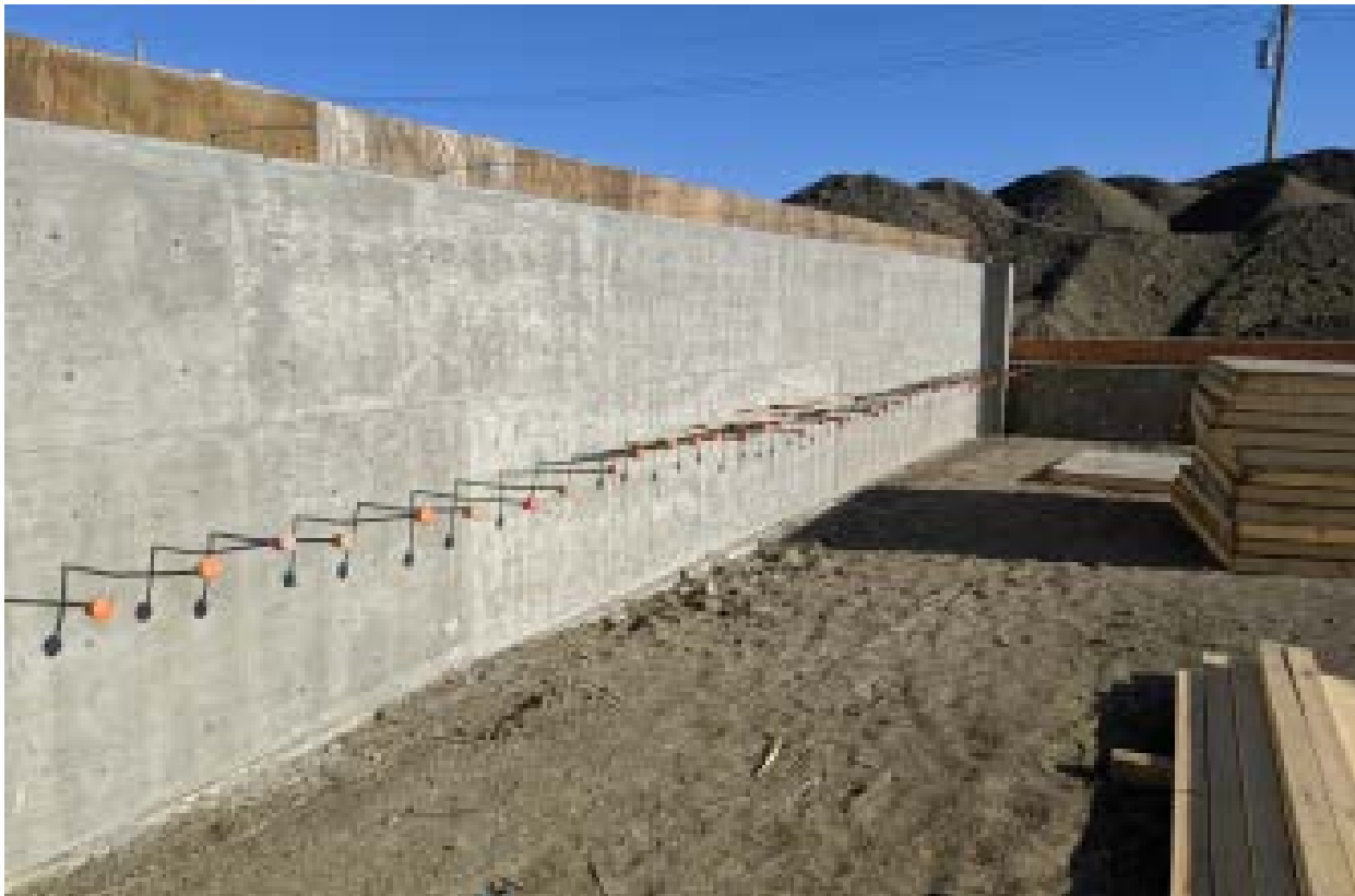
City of Raton RIP 00011 Solid Waste Convenience Center
