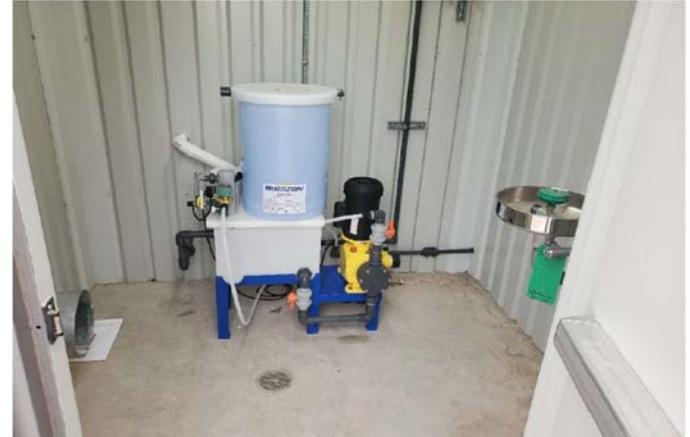
New water tank, booster station and chlorination system in Artesia
