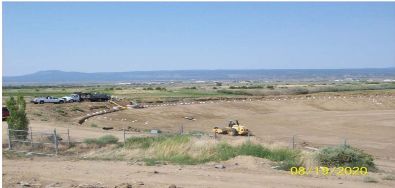
**Compaction of subgrade prior to liner installation.**
