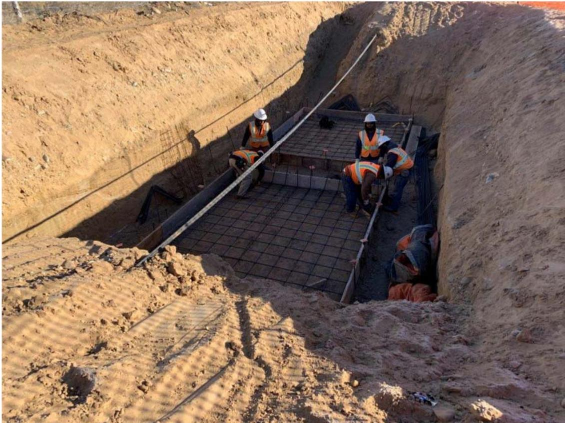
**Valley Water and Sanitation District Capital Outlay Project—Foundation for sewer lift station vault. Existing fiber optic line in the picture was relocated.**
