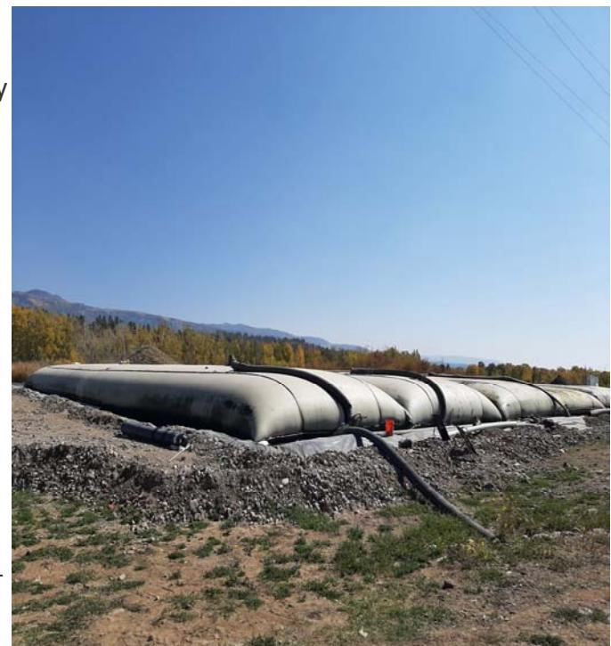
**Chama CWSRF 066 Geotubes for dewatering sludge from old lagoon**
