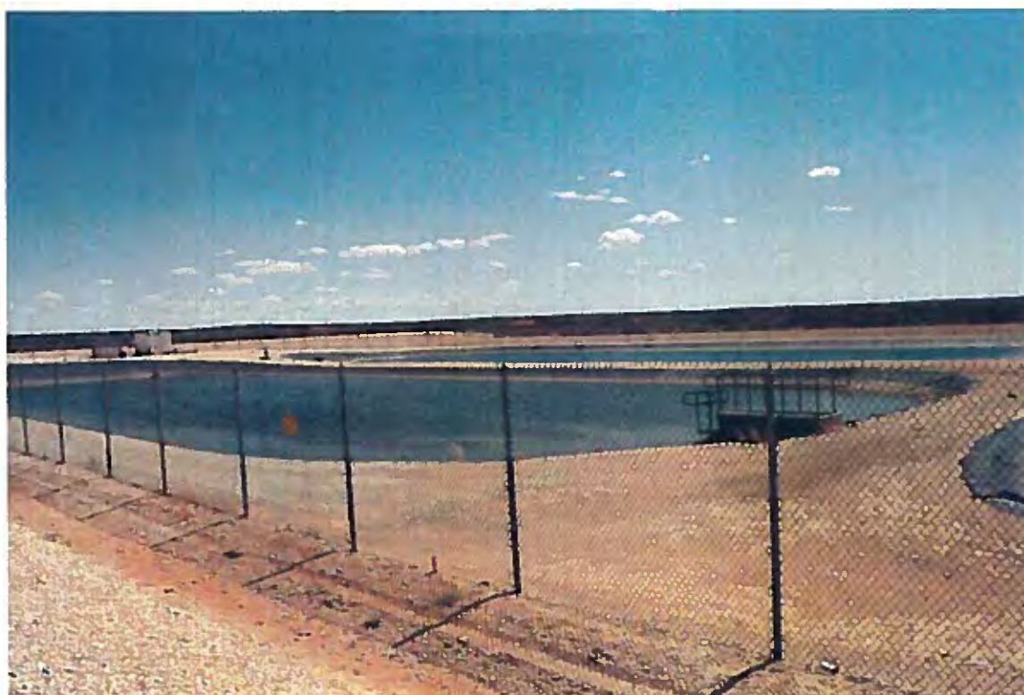
Unlined final evaporation cell
