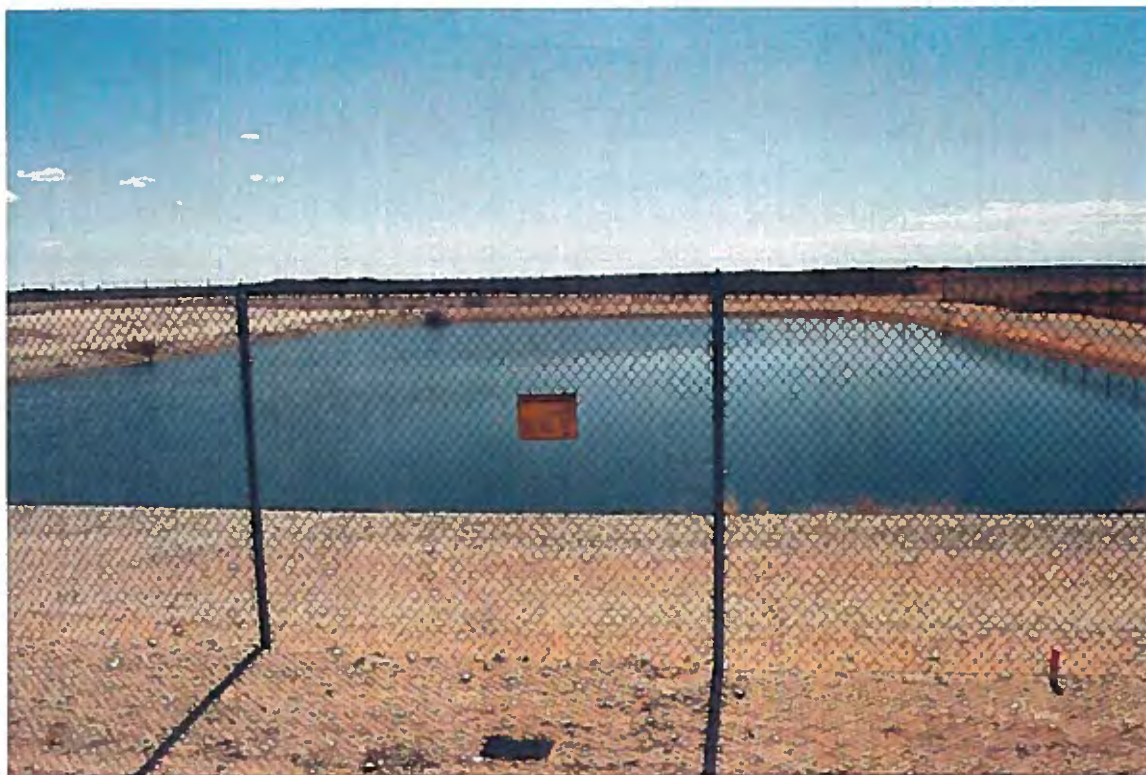
Unlined final evaporation cell
