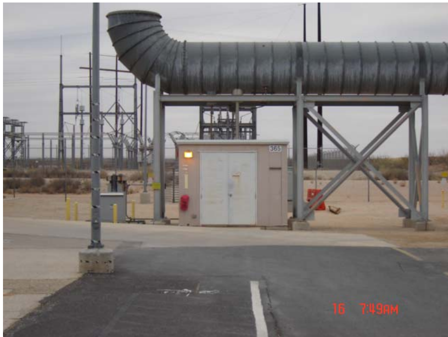
Figure WEA72-2. A view of Station B from the west.
