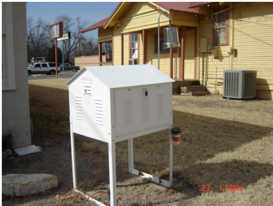
Figure WPL74-1. Low Volume Air Station outside the Oversight Bureau office in Carlsbad.
