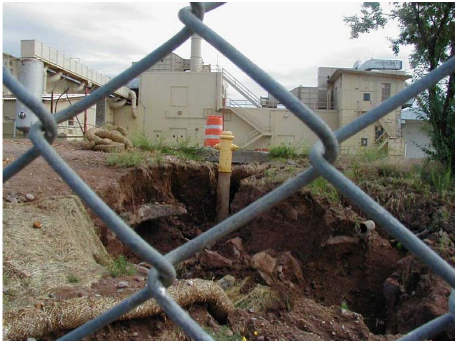
Figure LNP12-1. Erosion from July 5, 2008 release of 3.9 million gallon potable water at TA-21
