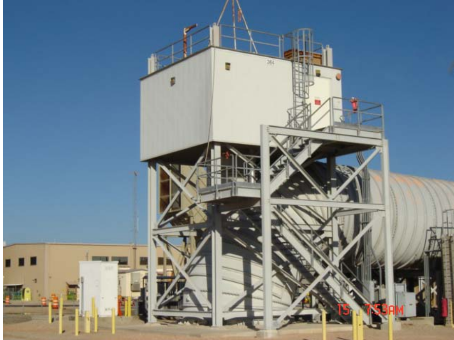
Figure WEA72-1. A view of Station A from the south-east.
