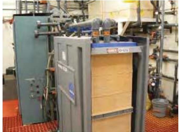
Figure 15.19 - Ionics Electrodialysis Reversal (EDR) Unit
