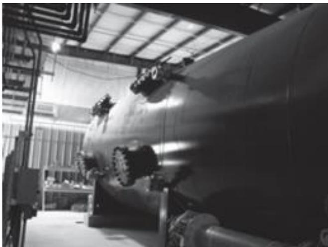
**Figure 15.2 - Biological Activated Carbon Absorber**
