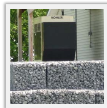
Elevated Emergency Generator
