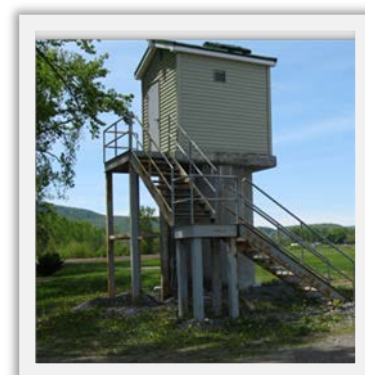
Wellhead above 100-year flood
