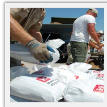
Sandbags to prevent intrusion of water
