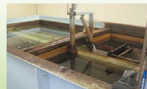
Drinking Water Treatment Plant
