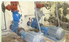
Booster Stations and Other Pumps
