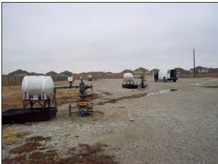
Figure 3.3-5. Site Documentation – Wells
