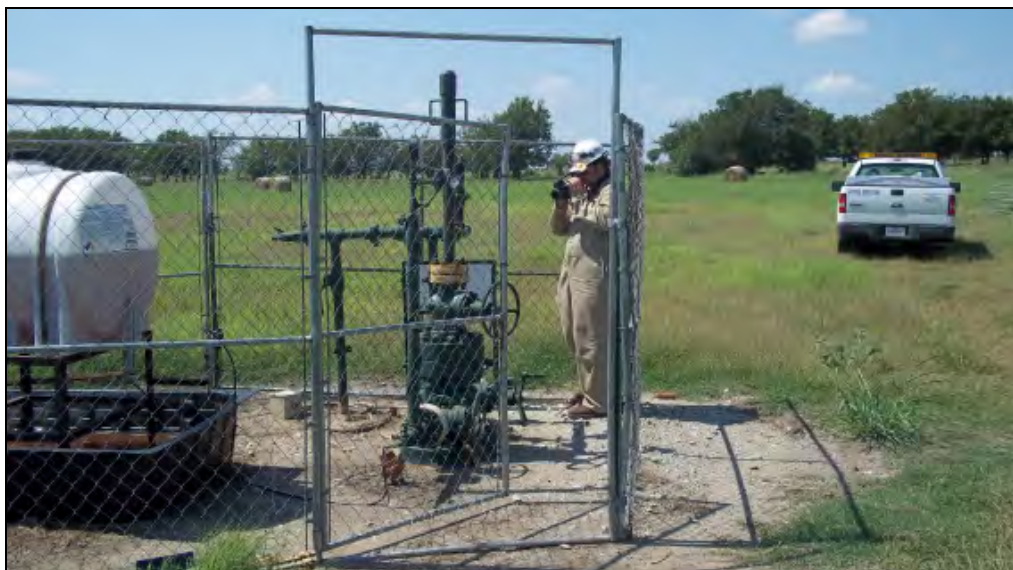
Figure 3.2-1. IR Camera Imaging at a Well Site
