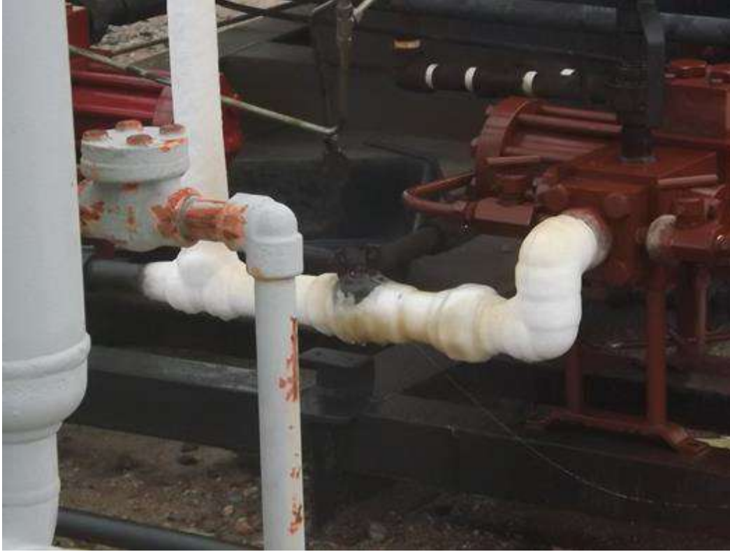
Figure S4. Photograph of the wet glycol discharge piping where the emission source was identified. The equipment was determined to be a Kimray 21020 PV model glycol pump. The maximum emission rate from the event was determined through interaction with the pump manufacturer and parameters recorded on-site.
